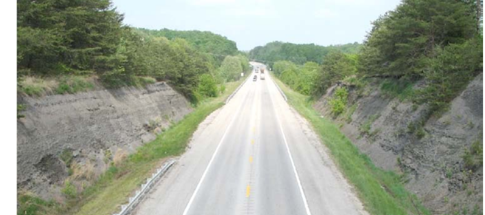
The Hal Rogers and Cumberland Gap Parkways and I-75 provide major transportation arteries for local industry. Photo by Dan Carey, Kentucky Geological Survey.
