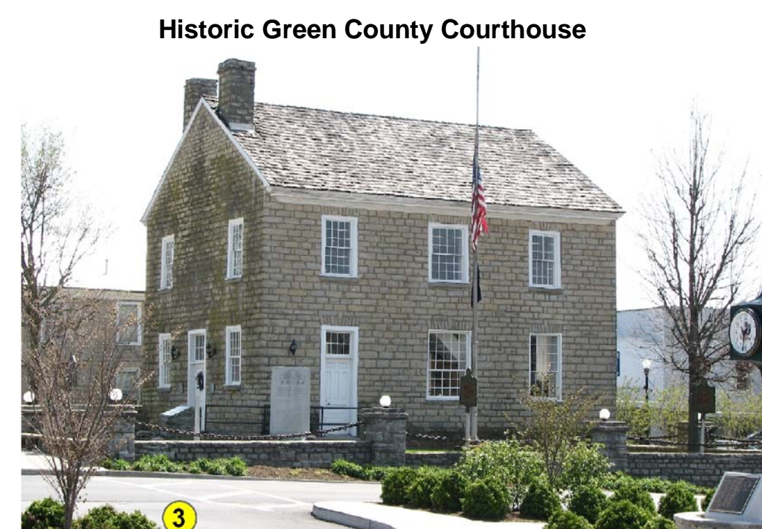
The former Green County courthouse, known as the oldest existing courthouse west of the Allegheny Mountains, was built of local limestone and completed in 1803. Green County, an area of 269 square miles in the Mississippi Plateau Region, was formed in 1793. The highest elevation, 1,045 feet, is less than a mile south of where Ky. 61 crosses the Lanes County line. The lowest elevation, 490 feet, is where the Green River leaves the county. The county population of 11,931 in 2000 was 3.6 percent greater than that of 2000. Photo by Dan Carey, Kentucky Geological Survey.
