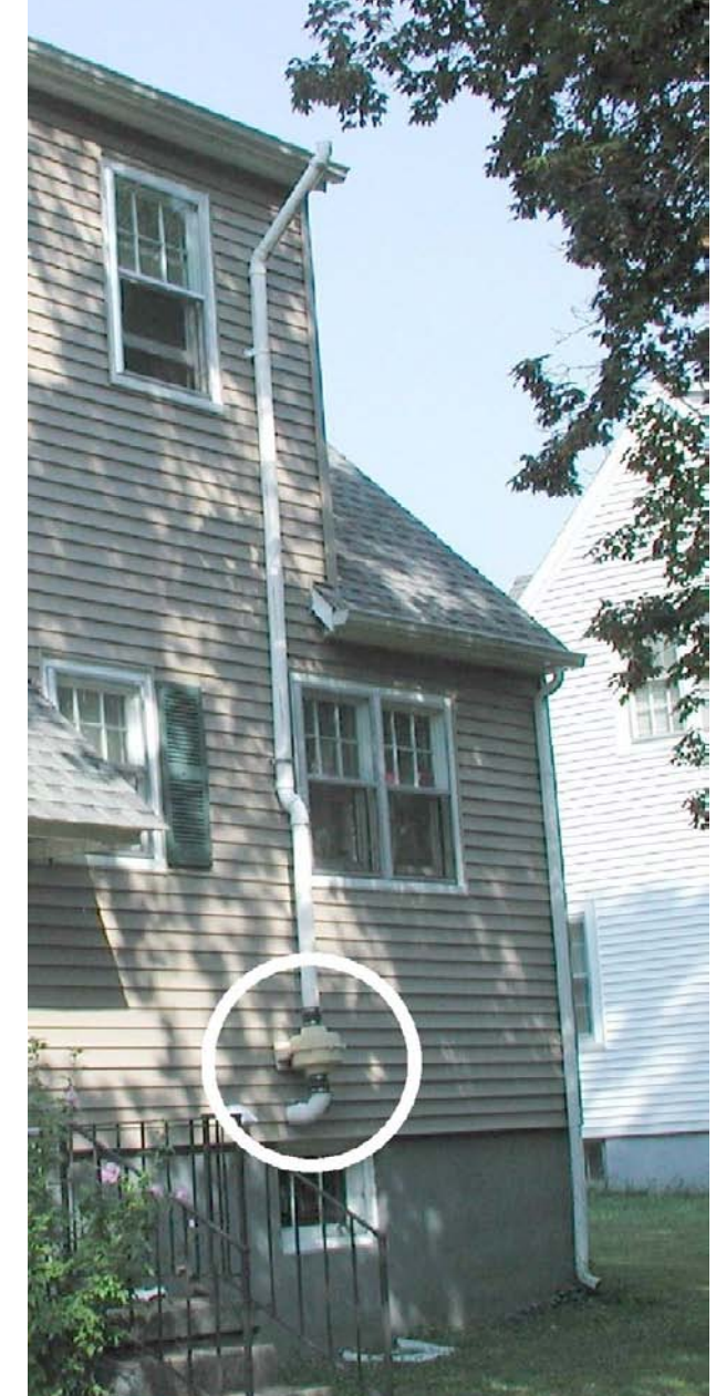
Ventilation system removes radon from the basement area of this home. Photo by Dan Carey, Kentucky Geological Survey.
