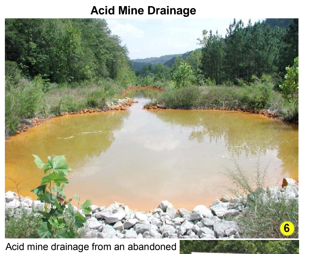
Acid mine drainage from an abandoned underground coal mine is exposed to limestone at this facility, reducing the acidity before it flows downstream. Photo by Randy Paylor, Kentucky Geological Survey.
