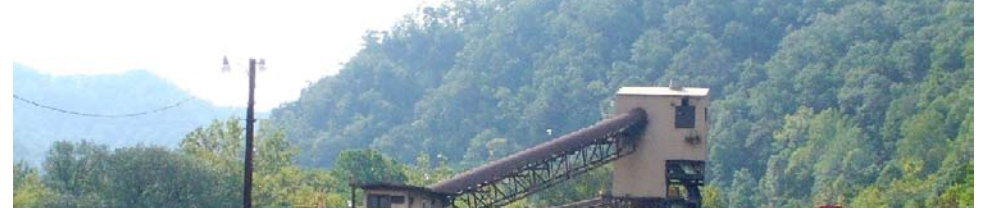
This coal tipple is a loading facility for coal trucks and trains near Fishtrap Lake. Photo by Bart Davidson, Kentucky Geological Survey.
