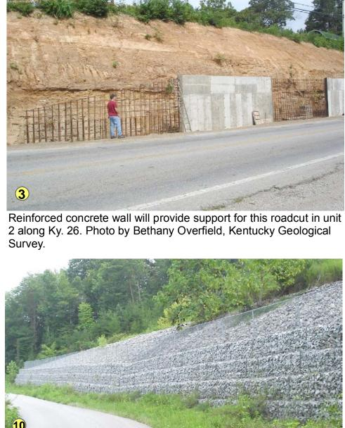
Rock gabions and a chain link fence provide stability to a cut slope in unit 2 along Doc Siler Road. Photo by Bethany Overfield, Kentucky Geological Survey.
