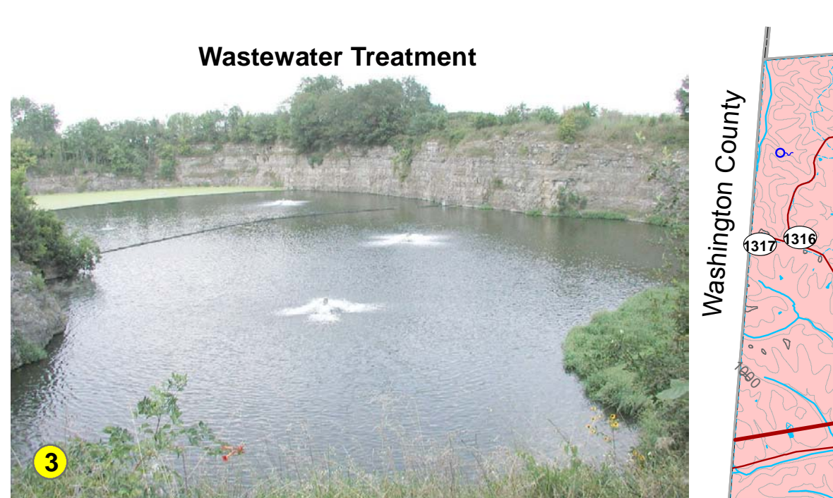
Wastewater Treatment Abandoned limestone quarry off U.S. 68 north of Perryville has been incorporated into the city's wastewater treatment system. Photo by Dan Carey, Kentucky Geological Survey.
