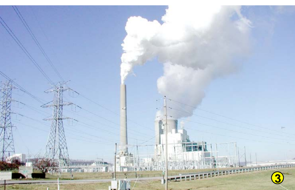
LG&E operates this 566 megawatt coal-fired power plant along the Ohio River just north of Wises Landing in southeastern Trimble County. Photo by Dan Carey, Kentucky Geological Survey.
