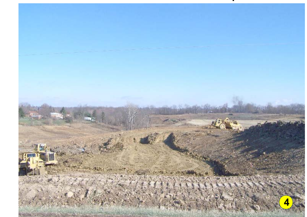
This area of new residential and commercial construction is located on Ky. 17 near Independence. Photo by Richard Smath, Kentucky Geological Survey.
