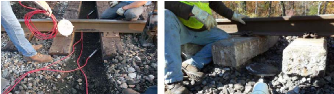
Figure 2.23 TTCI and Flatrock, KY In-Track Pressure Cell Installation
