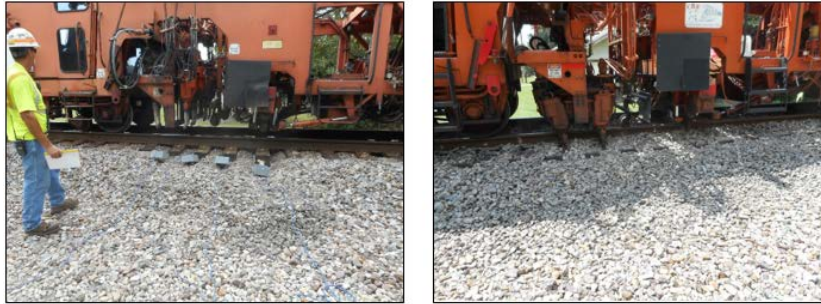
Figure 6.3 Tamping the Test Section
