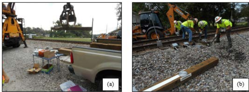
Figure 6.2 Handling and Placement of Instrumented Crossties
