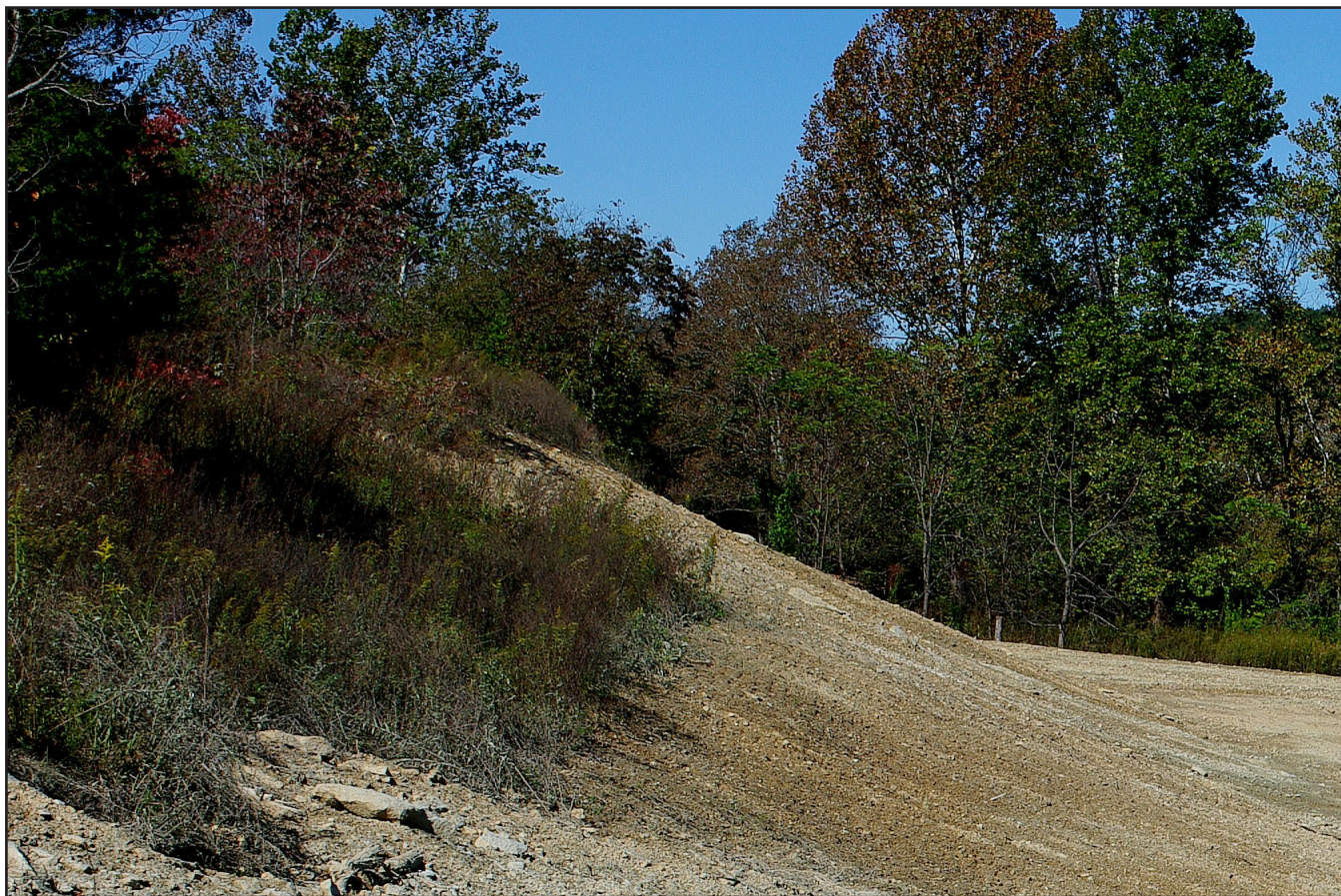
Figure 20. The well site was recontoured during remediation, as required by Hanson Aggregates, and obstructed with large stone blocks to hinder trespassing.
