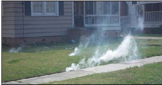
Smoke testing verifies leaks in sewer
