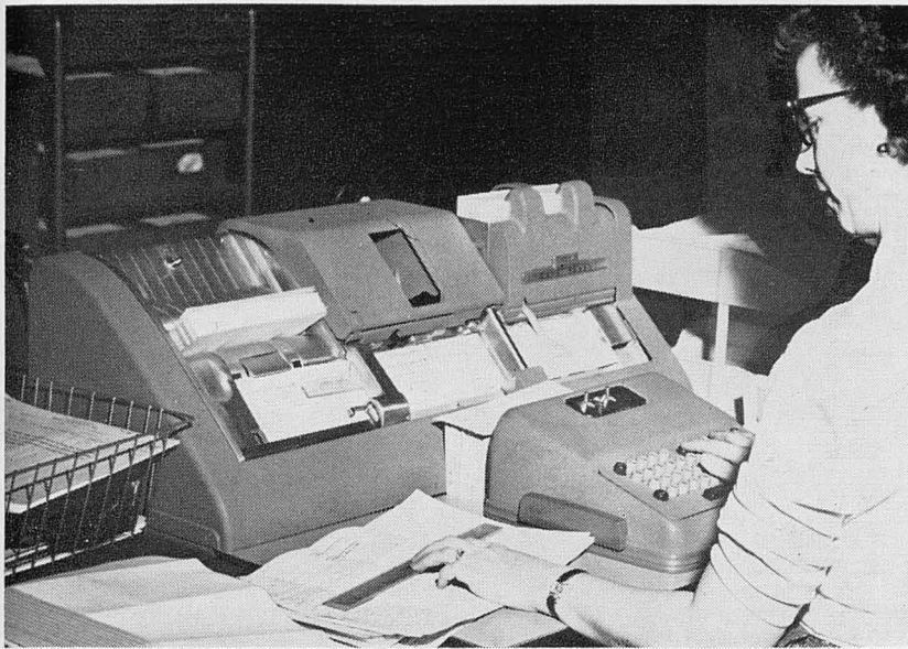
Figure 3.—IBM-024 (Key Punch). After the bids are opened the bid forms are taken to the key punch section. A key punch operator key punches information from the bid forms into cards. This information includes contractor's identification, unit bid, extension, and total bid.
