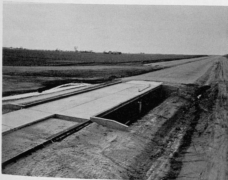
6. Four of 16 test bridge slabs.
