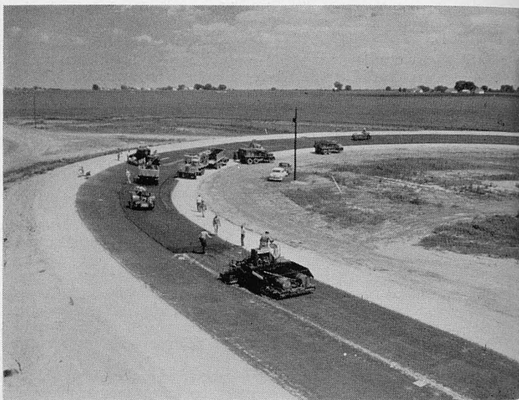
5. Flexible pavement operation.
