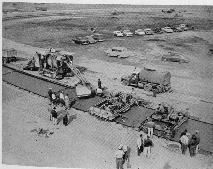
4. Concrete pavement operation.
