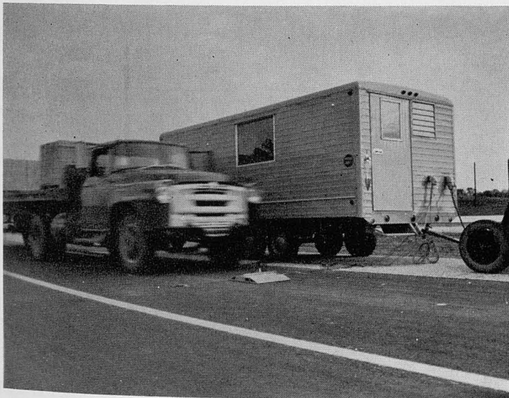
12. Test vehicle passing instrument van. Such vans contain instruments to measure deflections and strains under traffic.
