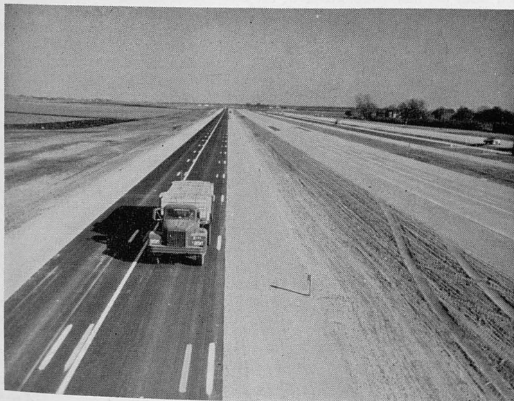
10. Test truck on flexible pavement tangent.
