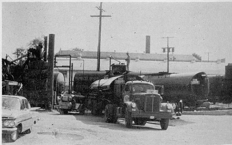
Fig. 4.—Truck trailer units loading for transportation of Curtiss-Wright binder to hot-mix bituminous plants. Note pilot plant digester at left of photograph.
