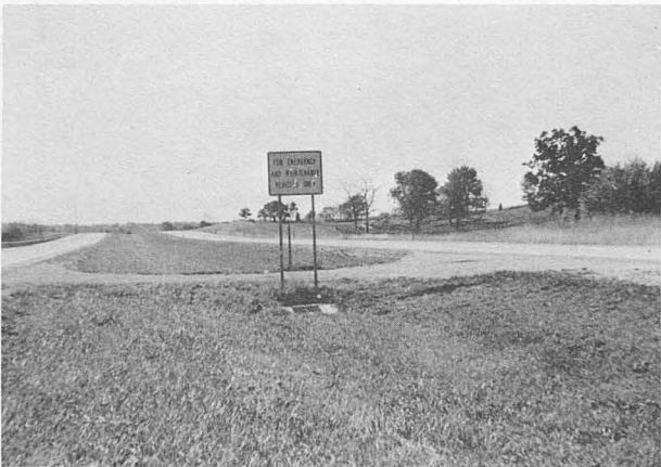
Figure 12. An objectionable mound created by a median crossover.
