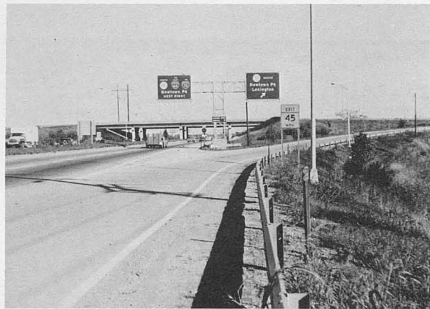
Figure 2. Unacceptable sign in gore area.
