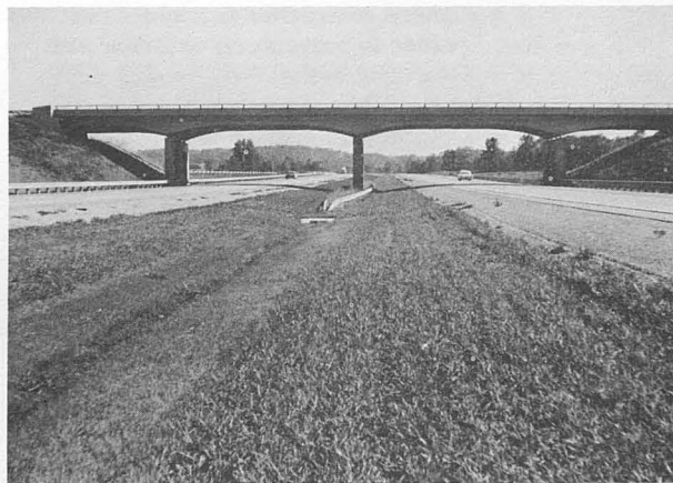
Figure 20. Guardrail protection at a median pier.
