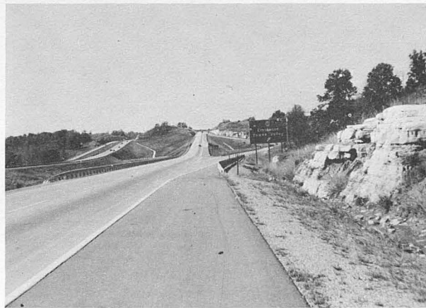
Figure 10. Continuous full-width shoulders carried over a structure.
