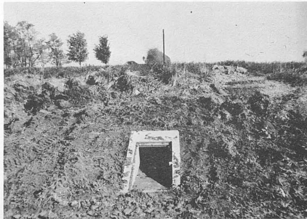
Figure 9. Traversable culvert entrance under construction.
