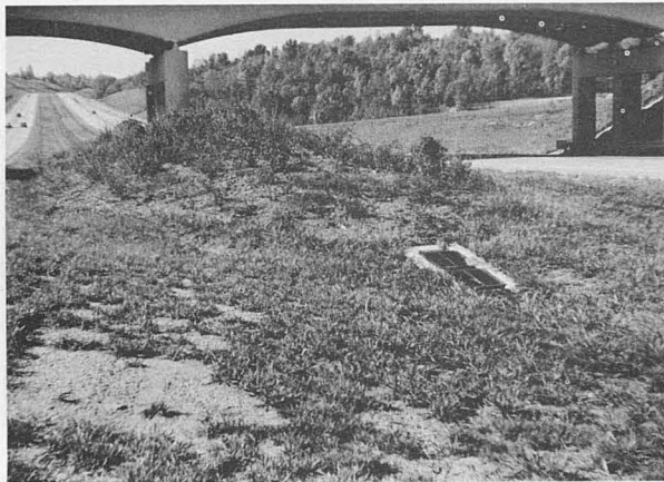
Figure 5. Traversable median drainage inlet at toe of earth berm.
