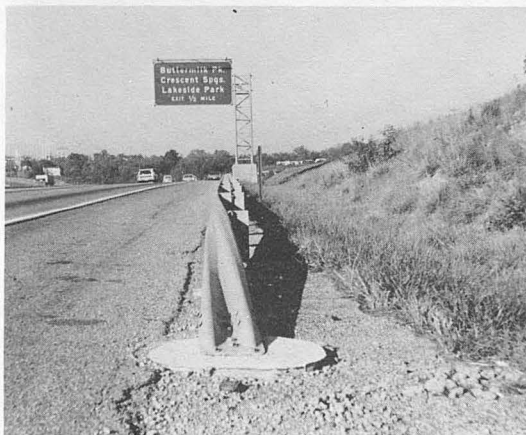
Figure 18. End treatment of guardrail.
