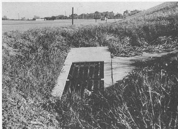
Figure 6. Cross drain in side ditch.
