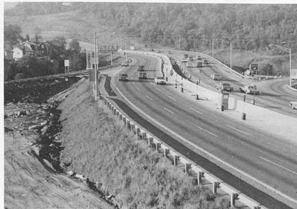
Figure 28. A rigid concrete median barrier under construction.
