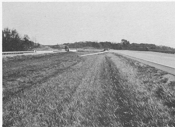
Figure 21. Guardrail protection at median opening.
