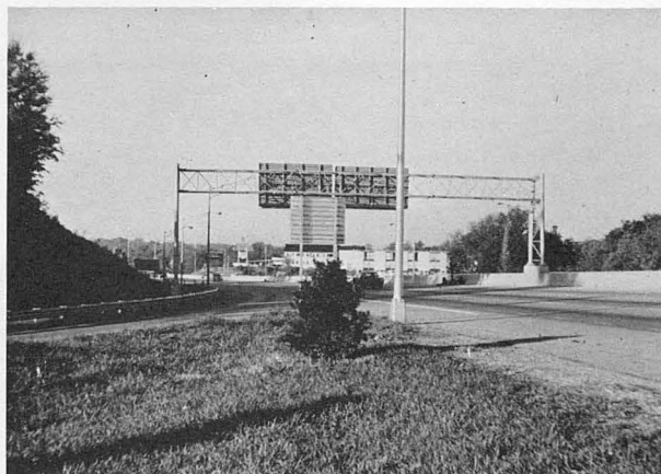
Figure 3. Exploitation of existing guardrail and median barrier installations in the location and design of sign supports.
