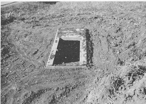
Figure 7. Cross drain in side ditch under construction.
