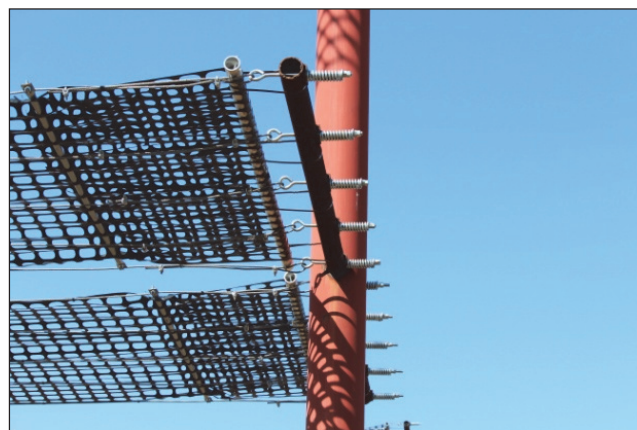
Figure 2. North crossbeam showing cable attachment with tensioning eye-bolt and spring assemblies. High-density, UV-stabilized snow fence material is strung between the support towers.
