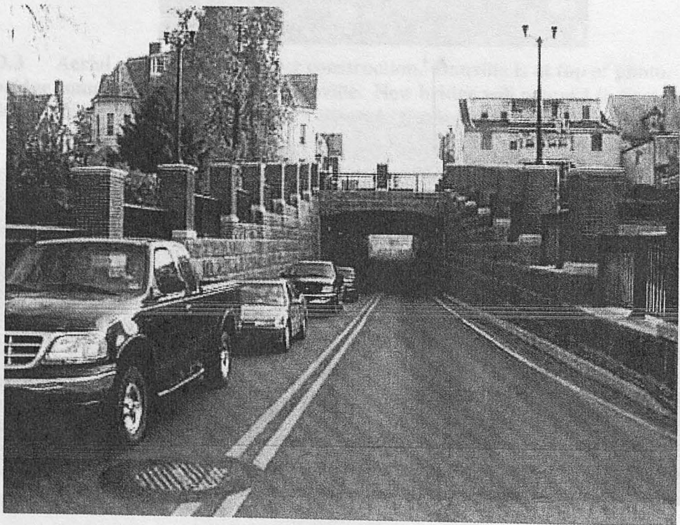
D.8 Entering tunnel from new bridge.
