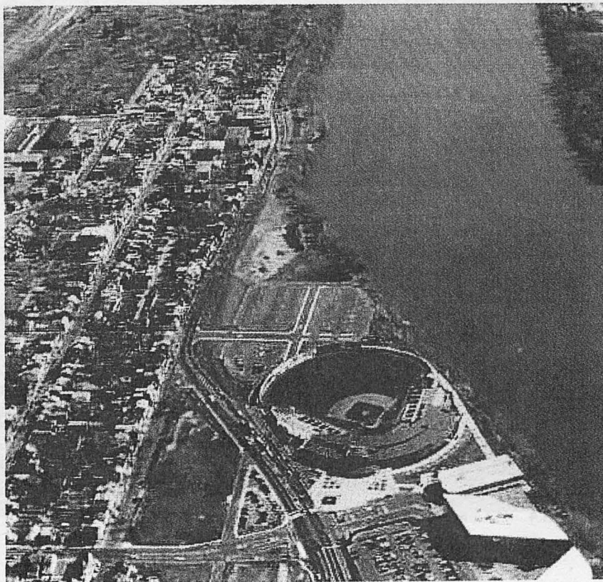
E.2 Aerial photo in Trenton. 2-lane section of Lambertson Road is in middle of photo.
