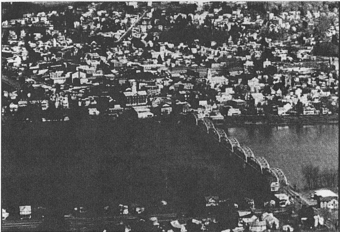
D.1 1904 Parker Through Truss Bridge from Riverside at lower right to Danville.
