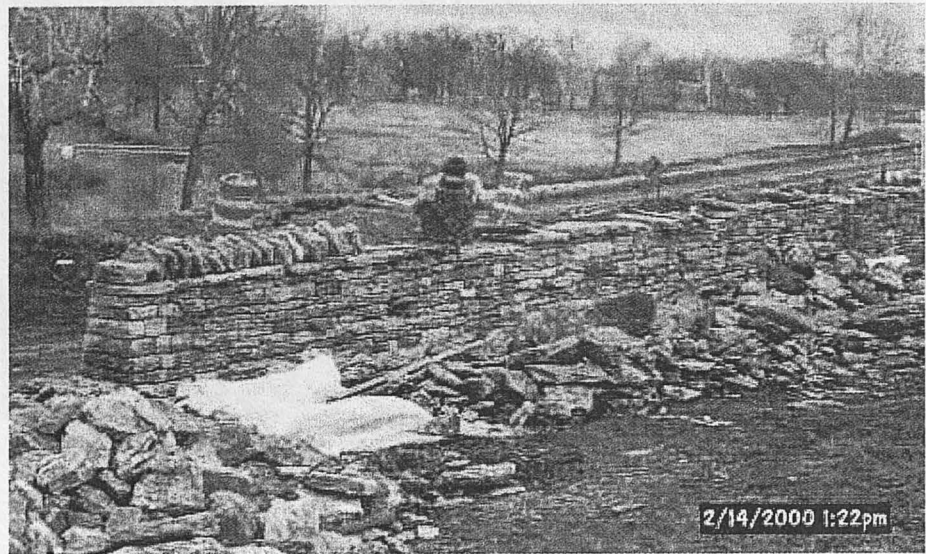
If not, stonewalls were dismantled and rebuilt
