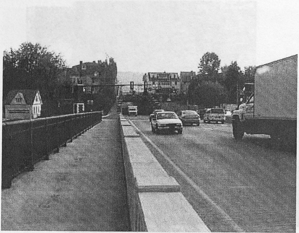
D.7 Photo taken from new bridge toward tunnel under Factory Street.
