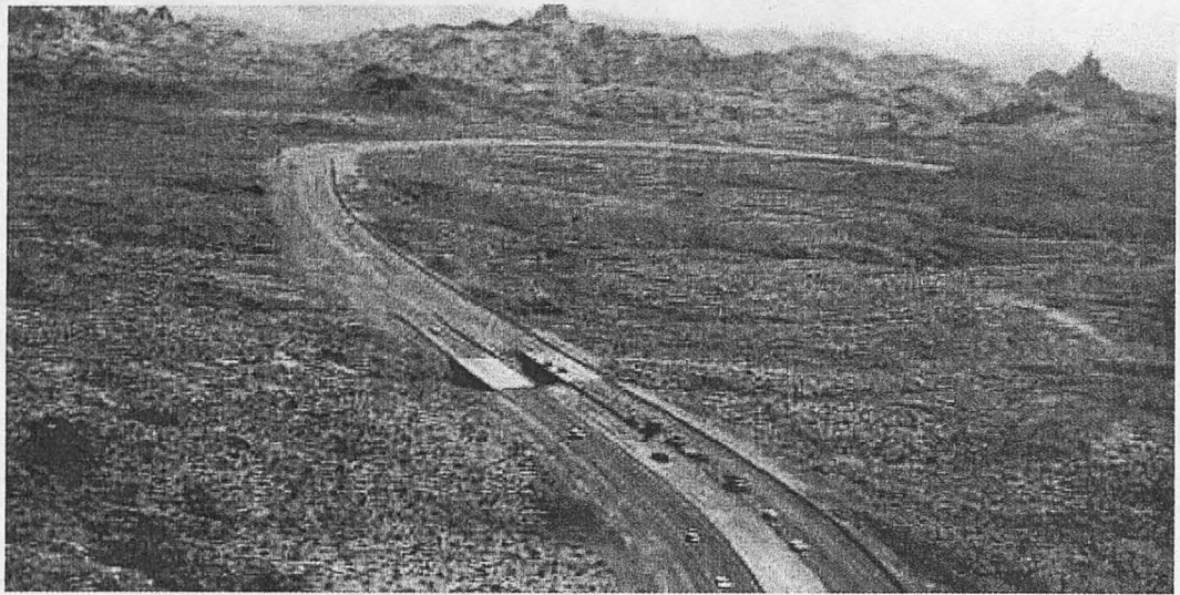
Construction of SR 68
