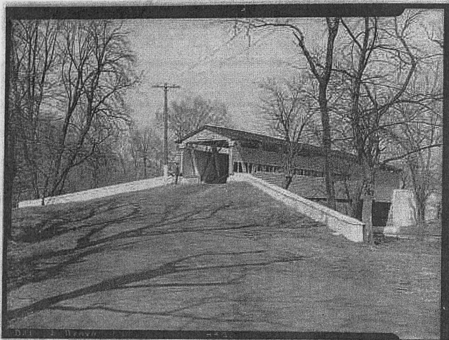
B.9 HABS Photo of Smiths Bridge constructed in 1839. Photo was taken from east approach in 1939.
