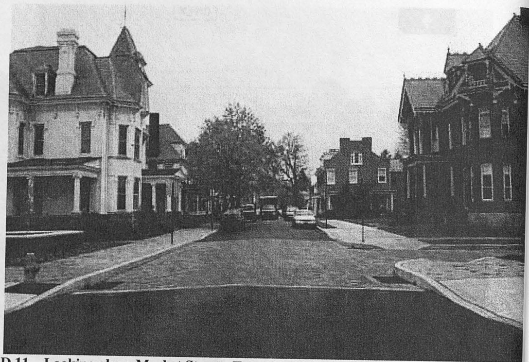
D.11 Looking along Market Street. Tunnel is below concrete brick pavers.
