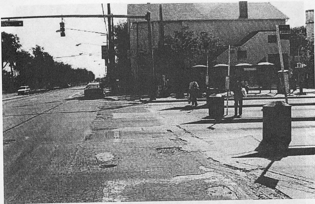
C.1 Mount Rainier before photo of bus shelter and bus holding lanes.
