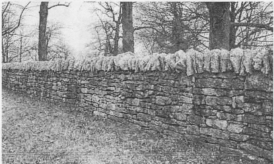
The roadway was aligned to miss historic mortar-less stone walls
