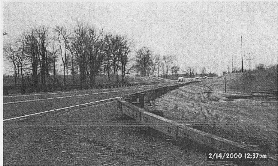
Steel-backed timber guardrail was used to provide driver safety while giving strong consideration to aesthetics
