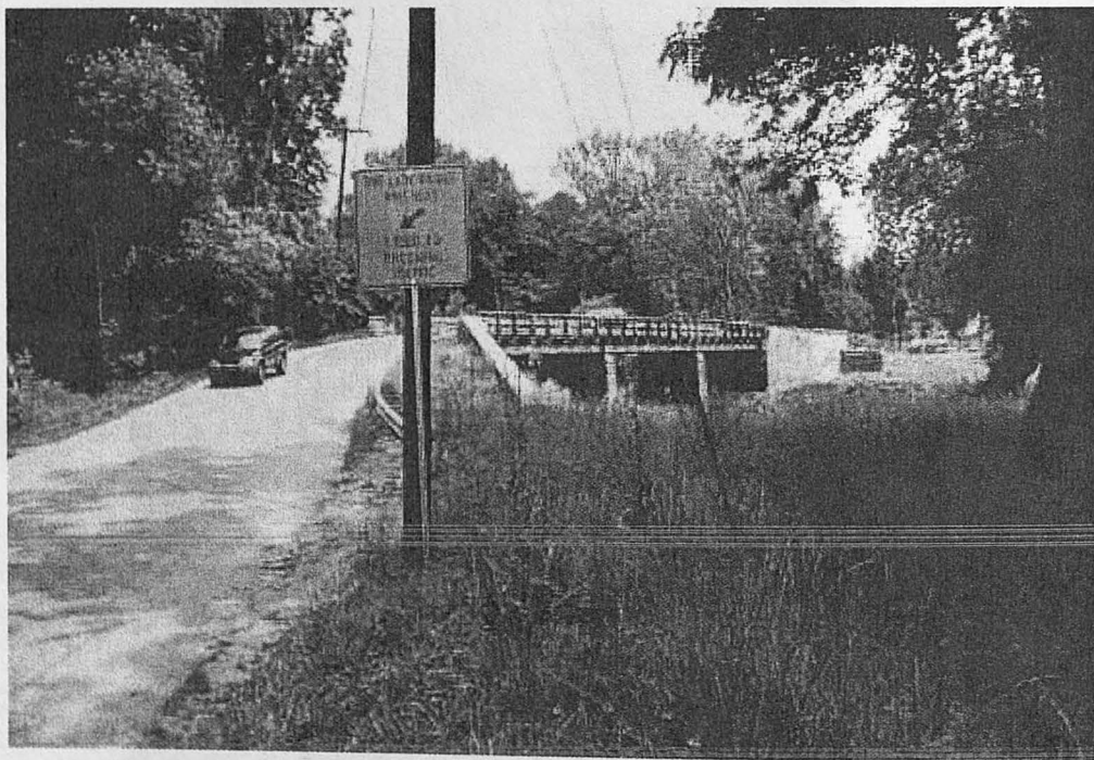
B.6 Smiths Bridge from west approach.
