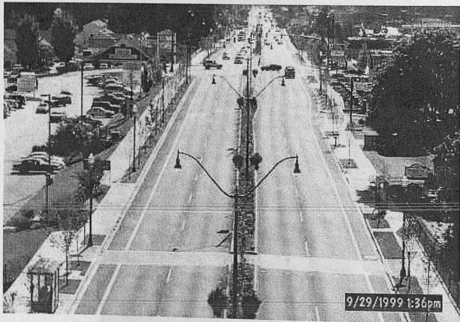
Figure 4. Bridgeport Way after, south view
