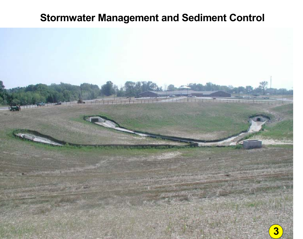
Soils exposed during construction are subject to high rates of erosion. The retention basin and pond in the background will trap sediment and prevent downstream water-quality degradation. Development is especially prominent along the main east-west connectors to Jefferson County to the west. Photo by Stephen Greb, Kentucky Geological Survey.
