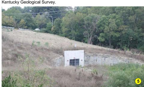
This outflow gate for the constructed underground drainage system shown in picuture 4b is located at the intersection of the East-West Connector and Collins Lane in Frankfort. The constructed underground drainage system exceeds 1 mile in length. Photo by Brandon Nuttall, Kentucky Geological Survey.
