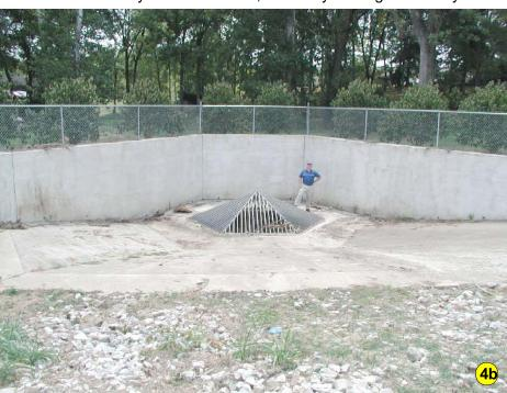
This constructed sinkhole at Hudson Hollow is adiacent to the natural sinkhole shown in picture 4a, and is used to control flooding during heavy rains. The underground system was built with two constructed swallets to redirect groundwater flow toward the Kentucky River. Photo by Brandon Nuttall,
