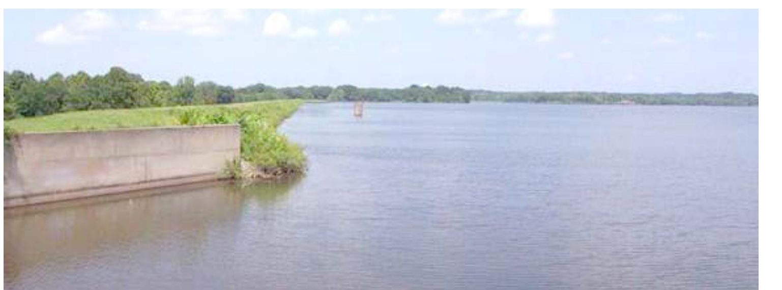
Lake Pee Wee is a 420-acre-lake constructed in the early 1950's to supply drinking water to the city of Madisonville. Currently, Lake Pee Wee provides drinking water to approximately 65 percent of the county. The lake holds 1.355 billion gallons of water and when necessary is recharged by pumping 9 million gallons of water per day from the Green River. Photo by Glynn Beck, Kentucky Geological Survey.
