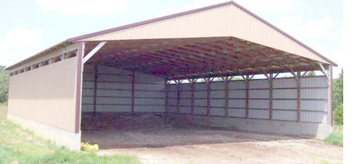
Poultry-litter storage buildings are used to assist farmers in meeting nutrient-management and water-quality guidelines set by the Kentucky Agriculture Water Quality Authority. Currently, approximately 150 chicken houses are in Hopkins County, and each poultry farm has at least one litter storage building. The above building is located on the Doug Brown Farm. Photo by Glynn Beck, Kentucky Geological Survey.
