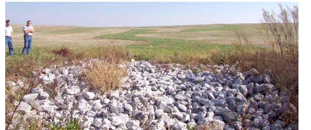
A typical way to control gully erosion, which is very common in Hickman County, is to construct a grassed waterway with a rock chute outlet. Funding for this structure is provided by the CRP CP-21 program through the USDA Conservation Reserve Program. Photo by Glynn Beck, Kentucky Geological Survey.
