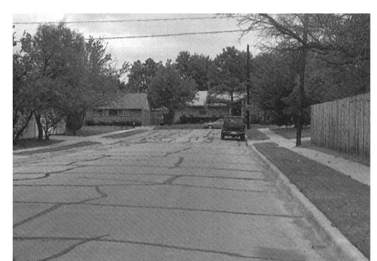
Paved roads constructed without precautions on swelling soils exhibit heaving, undulation, and extensive cracking. From AIPG (1993). (photo by Edward Nuhfer)
