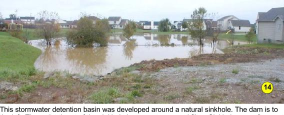
the left. The outlet throat of the sinkhole incorporates a sand filter. Sinkholes are often part of the natural flood detention system, and must be managed carefully to avoid creating additional flood damages as a result of development. Photo courtesy of Pattie Wilson, Versailles-Midway-Woodford County Planning Commission.
