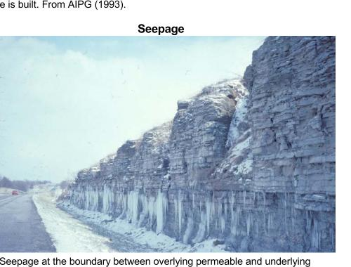
impermeable rocks. Often not evident during dry-weather construction, it can produce a variety of problems, including foundation disturbance, flooding, soil movement, wet basements, and failure of onsite wastewater treatment systems. These problems are common with construction on backfilled steep slopes. (photo by Paul Howell)
