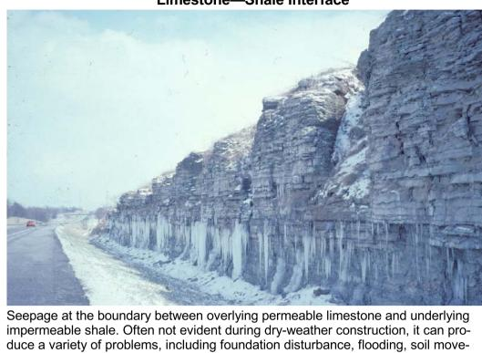
ment, wet basements, and failure of onsite wastewater treatment systems. These problems are common with construction on backfilled steep slopes. Photograph by Paul Howell, U.S. Department of Agriculture—Natural Resources Conservation
