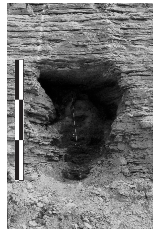
Figure 7. Small solution cave occurs on both sides of the cut, east is side shown here. The cave bottoms at the point where the fault meets the Fairview–Grant Lake Limestone contact, and is filled with silty clays and silts. White segments approximately 10 cm.
