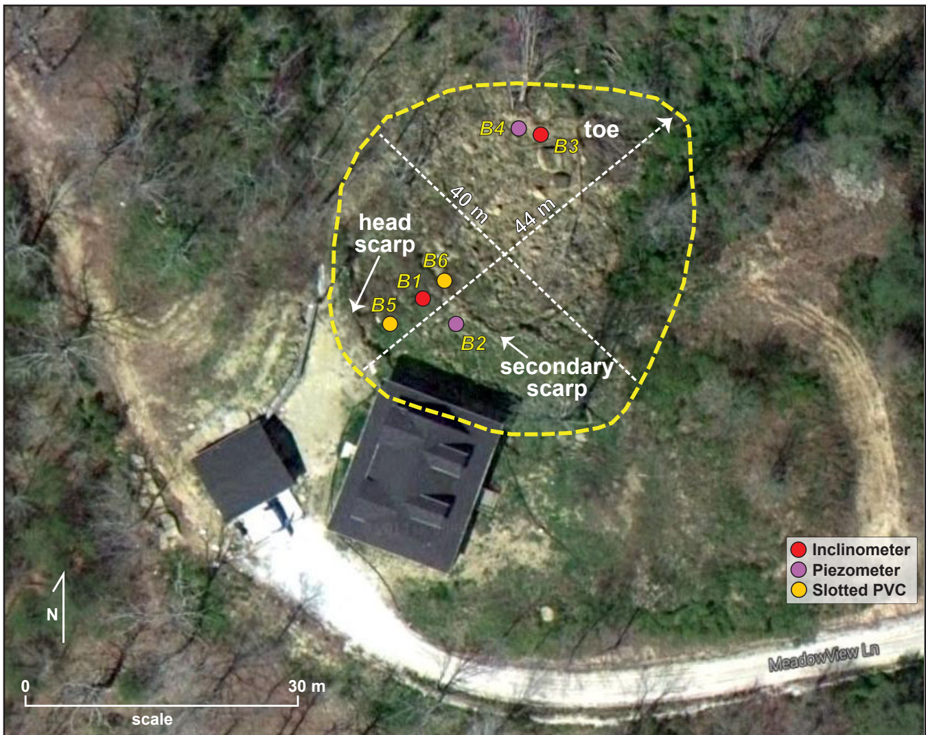
Figure 3. Aerial image of the Meadowview landslide. The main landslide area is within the dashed outline. Axes show dimensions of the slide. Borehole locations and instrumentation types also shown.
