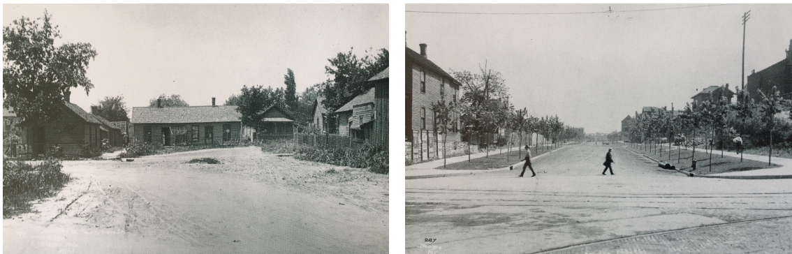
Figure 7.4, left No date, black-owned residences before demolition for Kansas City’s boulevard, the Paseo . Both photos courtesy of the Kansas City, Missouri, Parks and Recreation Department Archives. Figure 7.5, right No date, the Paseo after resident-displacement, built to improve urban walkability and greenspace .
