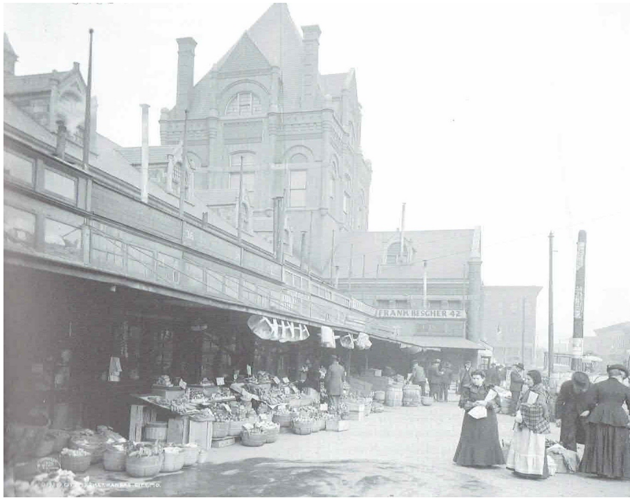
Figure 2.12 City Market, 1906. Photo from Missouri Valley Special Collections, Kansas City Public Library.
