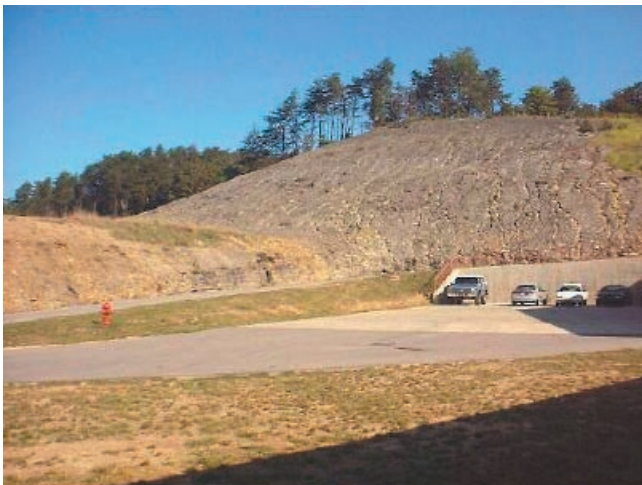
Figure 5. Chattanooga Shale outcrop behind the middle school (toward the north). Note retaining wall.
