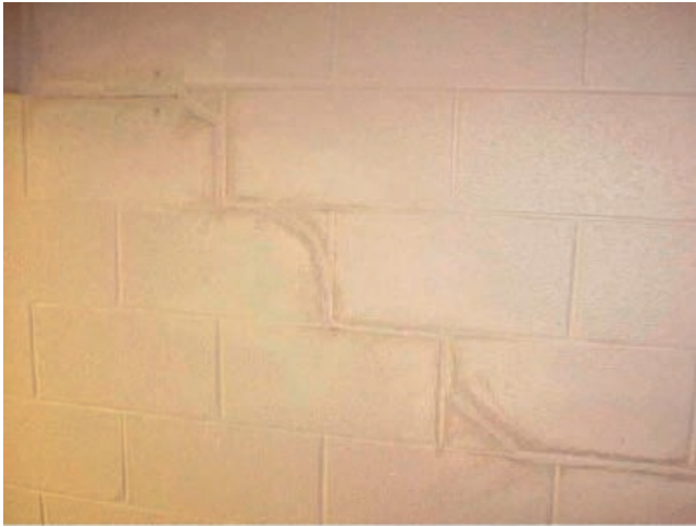
Figure 13. Repaired masonry block cracks.
