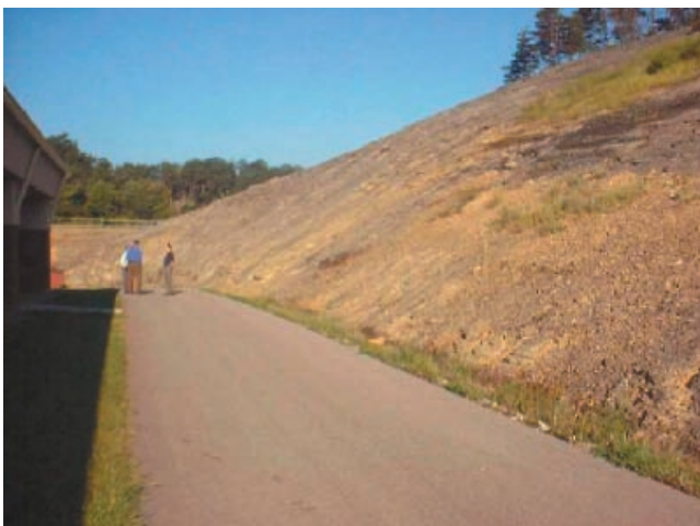
Figure 6. Outcrop and road behind Estill County Middle School.
