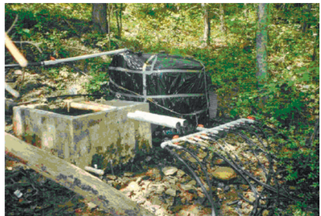
Figure 2. Nonregulated mine-water distribution system. Water is transported into a large cistern equipped with a 12-valve manifold; each individual supply line leads to one or more households. The cistern is covered with black plastic to block sunlight and control algae growth. Overflow at the top of the cistern prevents freezing in winter.
