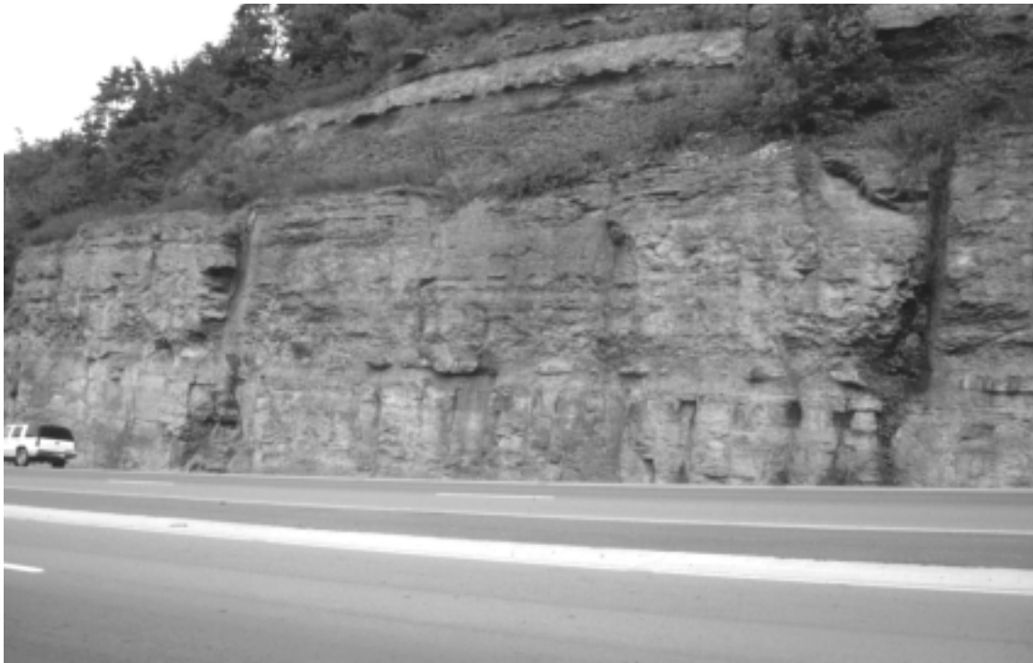
Figure 8. Fracture zone along Ky. 80 roadcut identified by Landsat TM lineaments (looking east).
