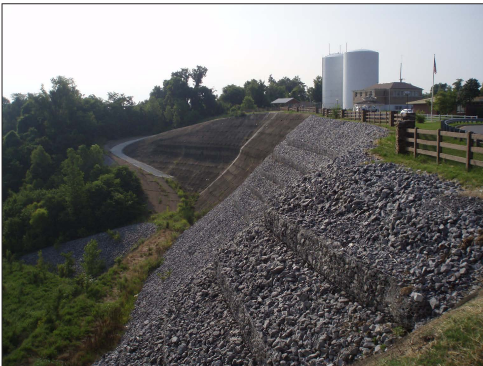
Figure 2. Repaired landslide in Hickman, Fulton County.
