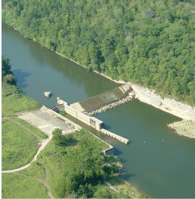
Figure 2 Aerial Photograph of Lock and Dam No. 8
