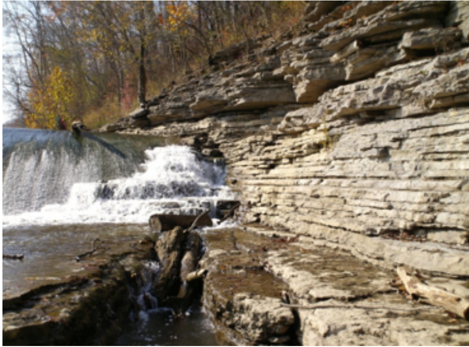
Figure 10 Geologic Reconnaissance – Highwall and Benches Downstream Along Left Abutment
