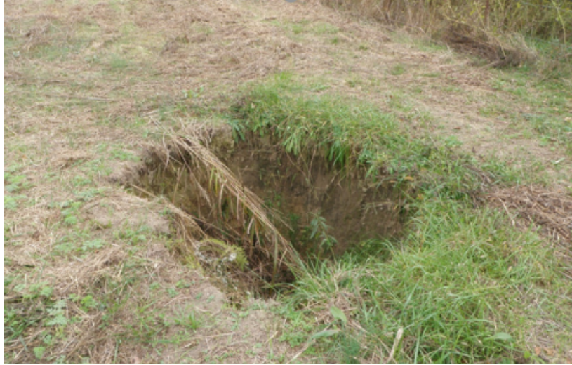
Figure 8 Sinkhole Observed Near the Site Entrance
