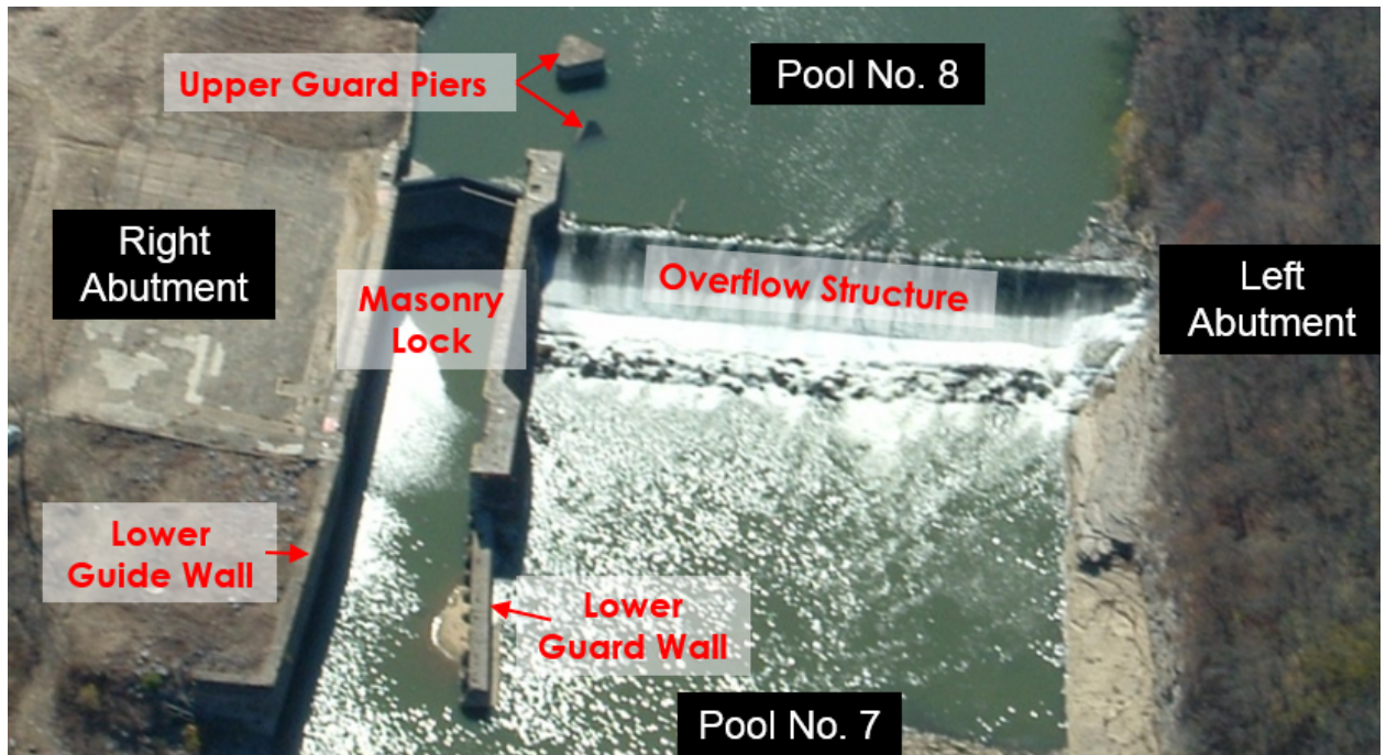
Figure 3 Lock and Dam No. 8 Site Features
