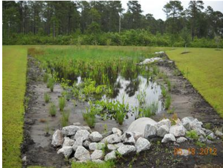
Figure 3.2. Typical of a Stormwater Wetland
