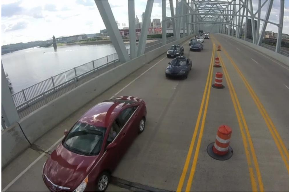
Figure 10 Snapshot from video of zipper merge in action on Taylor Southgate Bridge
