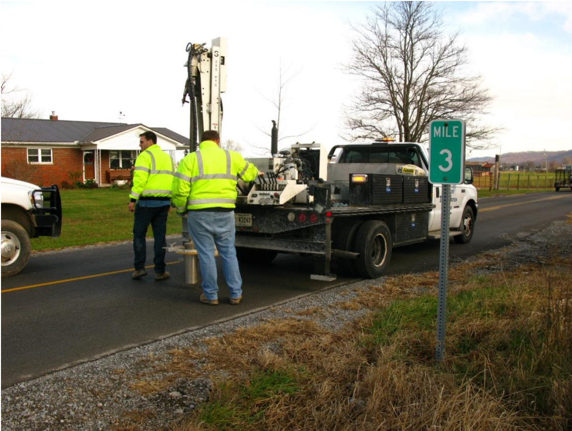
KTC Crew Coring Roadway for FDR Sample.
