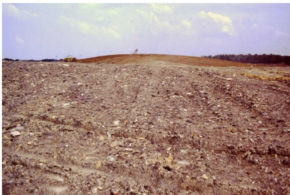
Fig. 143. Coal mine reclamation in the Western Paradise Coalfields (A. D. Karathanasis).
