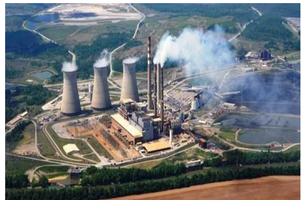
Fig. 144. Aerial view of the coal-fired Power Plant operated by TVA in Muhlenberg County, Kentucky (KGS).
