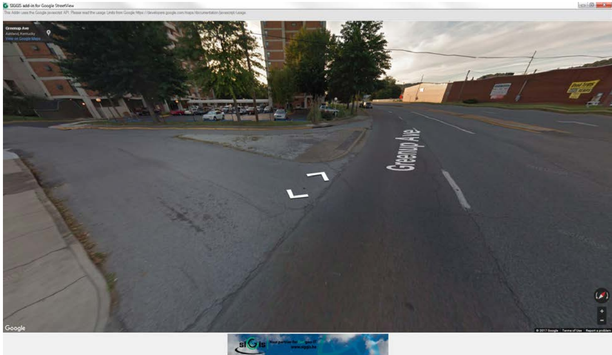
Figure 27: Paved Auxiliary Facility without Detectable Warnings (PresenceAF=1, RampAF=1)
