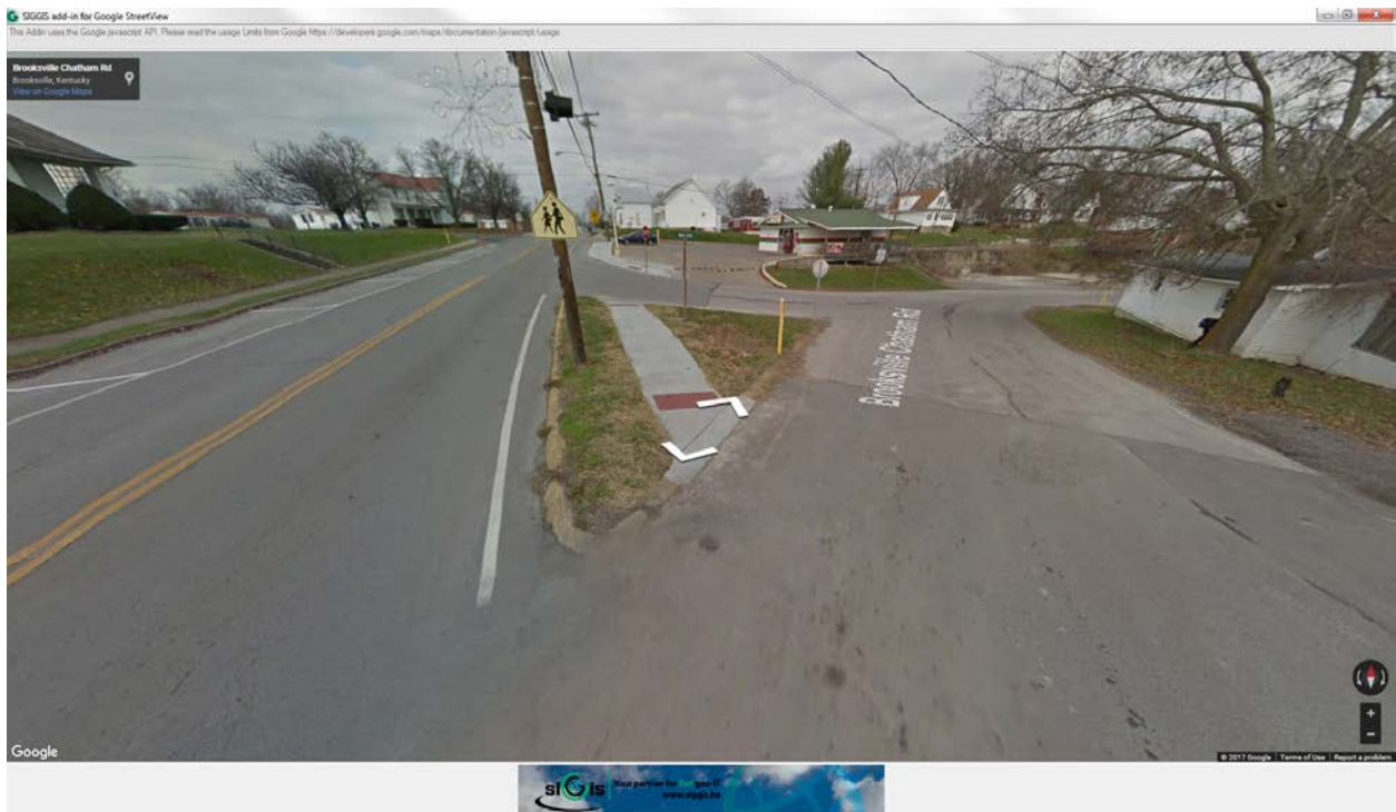
Figure 26: Paved Auxiliary Facility with Detectable Warnings (PresenceAF=1, RampAF=2)
