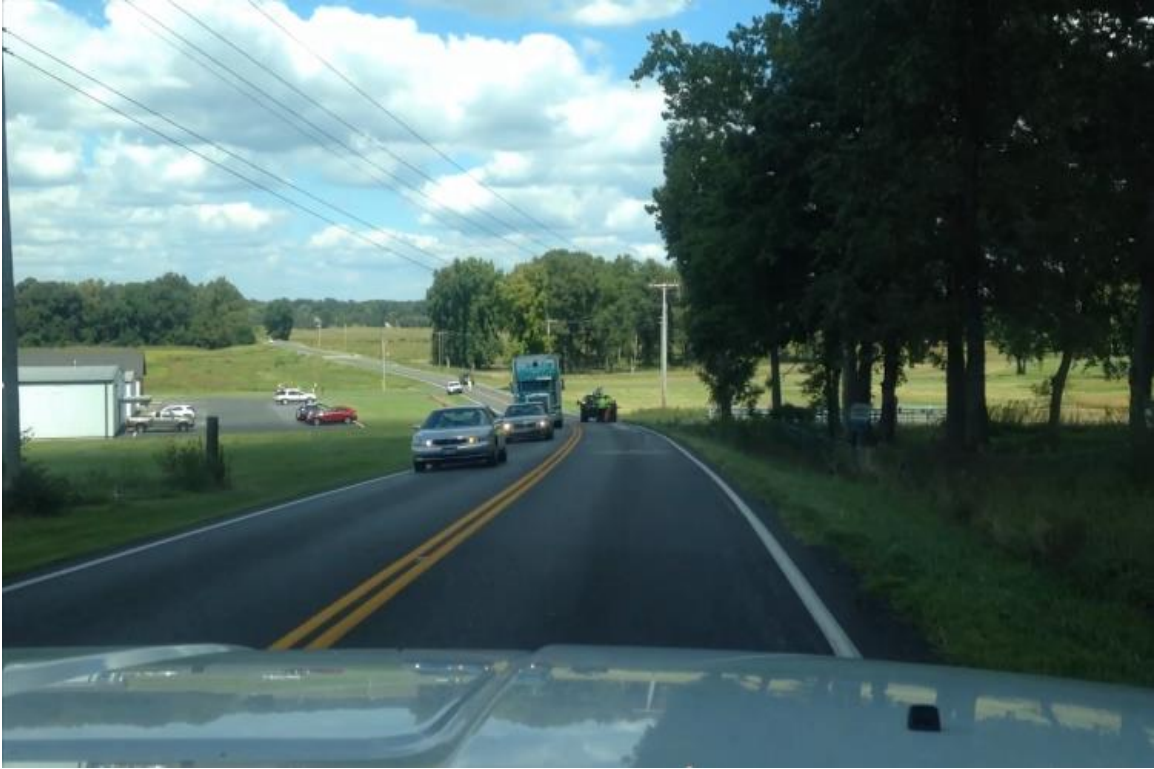
Figure 10 US-641 Calloway County project site
