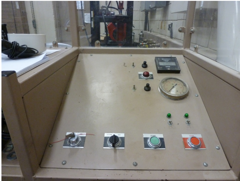
Figure 4-15 Hydraulic press control table
