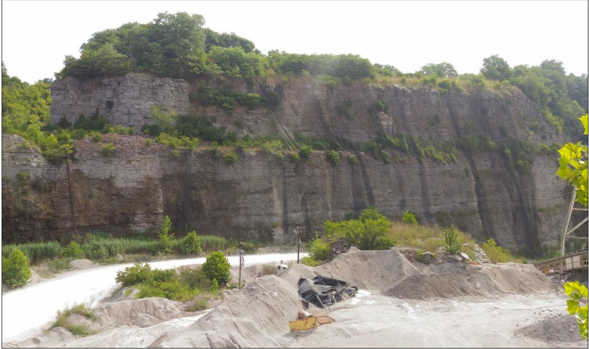
Figure 1-3: High-wall under study at Nally & Gibson, Limestone Quarry, Georgetown, Kentucky
