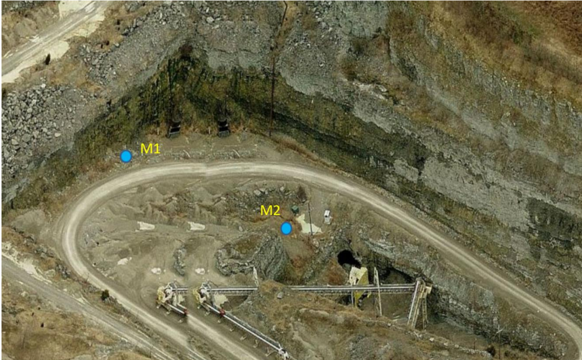
Figure 3-2: High-wall under study at Nally & Gibson, Limestone Quarry, Georgetown, Kentucky
