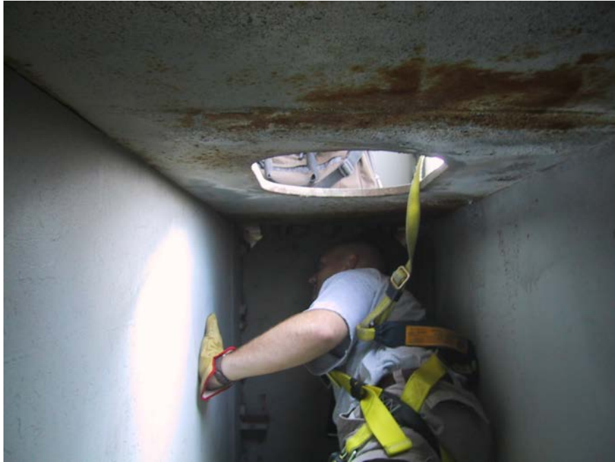
Figure 12 Good visibility is necessary for visual inspection
