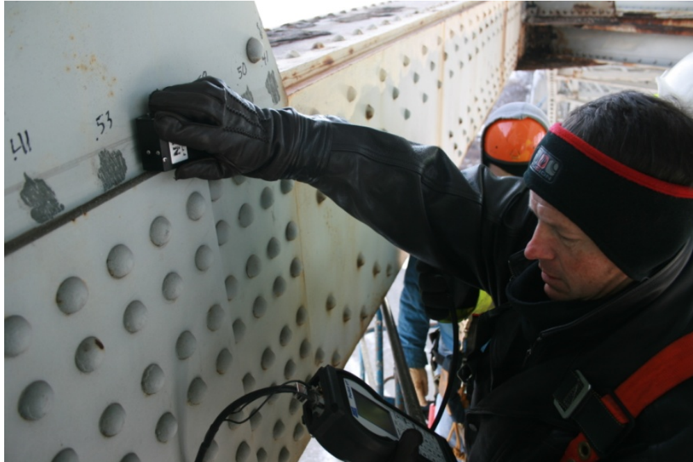
Figure 40 Use of ultrasonic thickness gage to inspect a gusset plate (Weir, W.R., “Methodology in Gusset Plate Inspection, Evaluation & Rating,” Transystems Presentation at the Midwest Bridge Working Group Fall Meeting, December 10, 2008).
