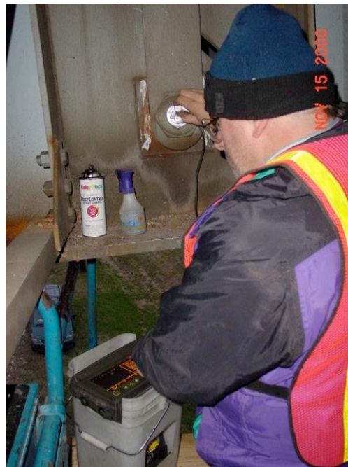
Figure 32 Typical ultrasonic pin inspection (Indiana Statewide Pin And Hanger Inspection Program – Final Report Indiana Route 237 over Ohio River Cannelton, Indiana, Bridge No. 237-62-06512 A, Prepared for the Indiana Department of Transportation by Wiss, Janney, Elstner Associates, Inc., November 15, 2000)
