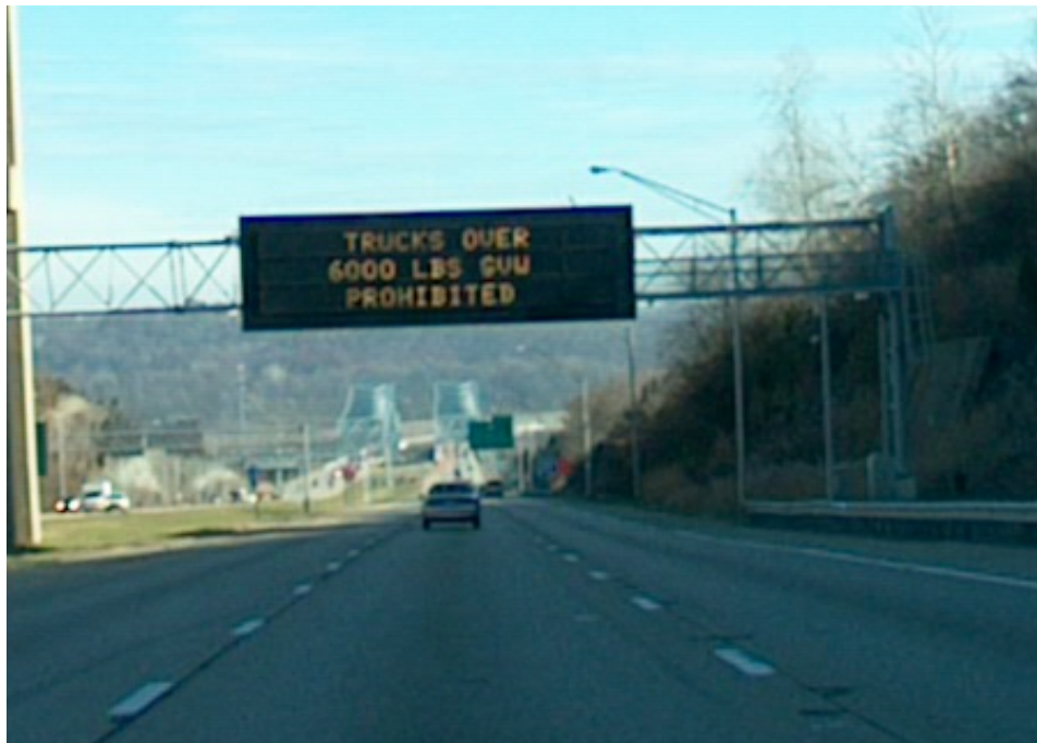
Figure 4 I-275 Northbound bridge over the Ohio River temporarily posted at 6,000 lbs for trucks due to a cracking problem in 2008
