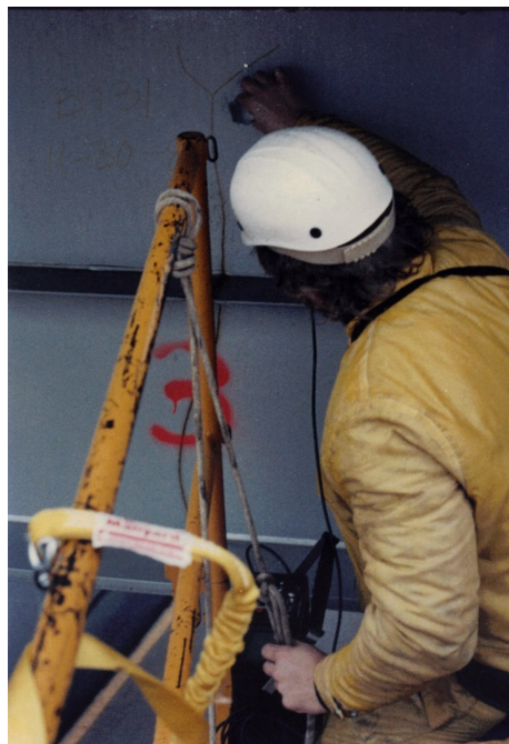
Figure 57 Major crack in fascia girder of the KY 117 bridge over I-24 in 1987
