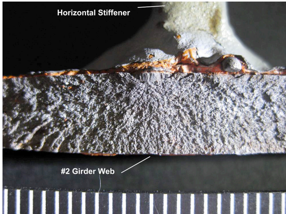
Figure 55 Fractured girder web with fracture origin (arrow) and surrounding fast (cleavage) fracture that severed the web (millimeter scale at bottom of picture)
