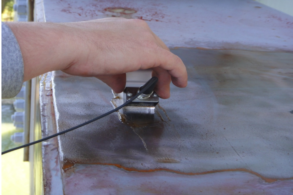
Figure 37 Shear wave UT of a butt-weld using an angle-beam transducer on I-275 Carroll Cropper Bridge
