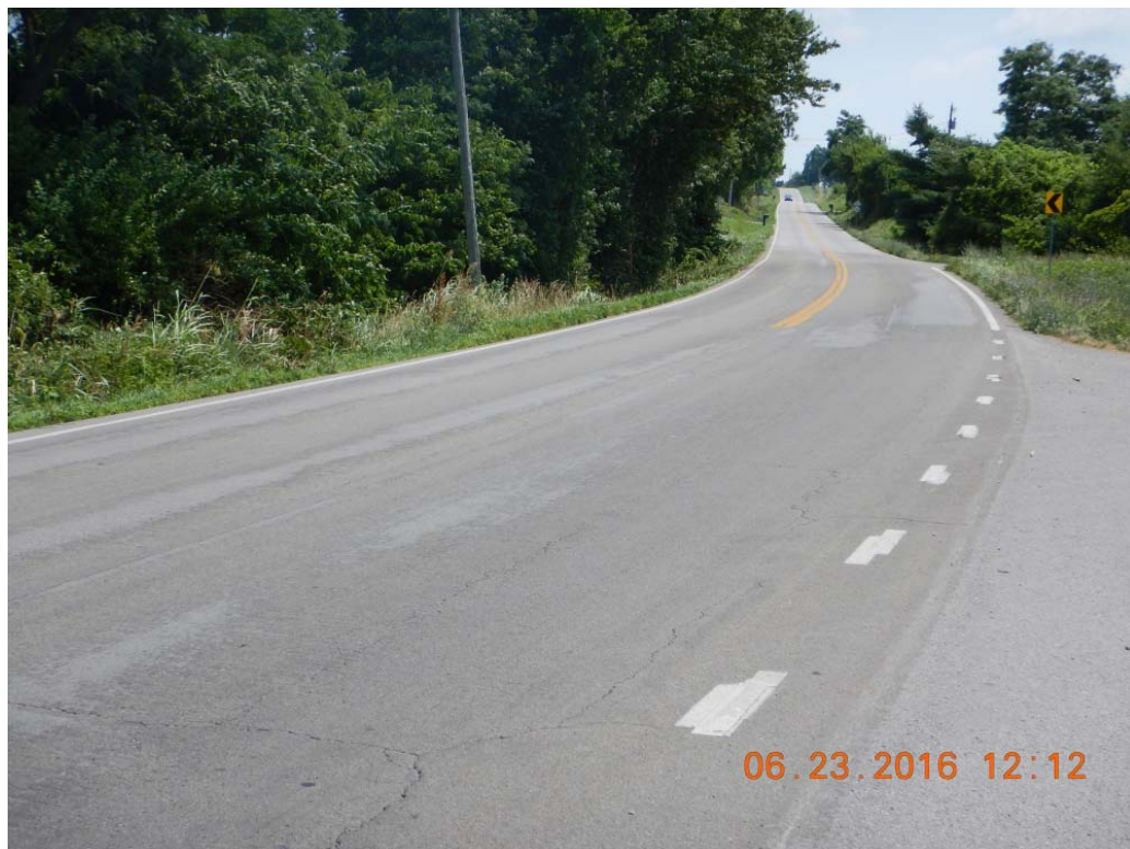
Figure 7.12: Boyle County, Surface Wearing, Microsurfacing
