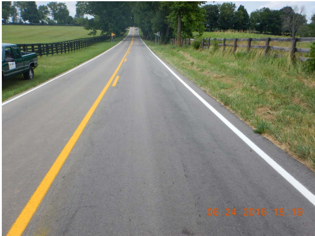
Figure 7.13: Fayette County, Surface Wearing, Microsurfacing
