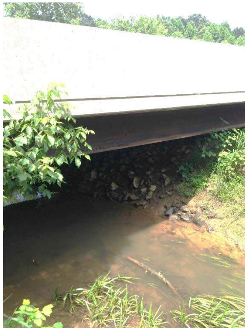
Figure 26. Low Water Clearance UWS Bridge on KY 6 in Knott County
