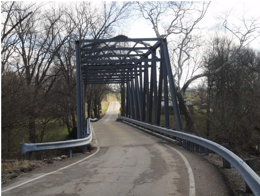
Figure 28. Painted Truss Employing Weathering Steel KY 3364 Bridge in Bourbon County
