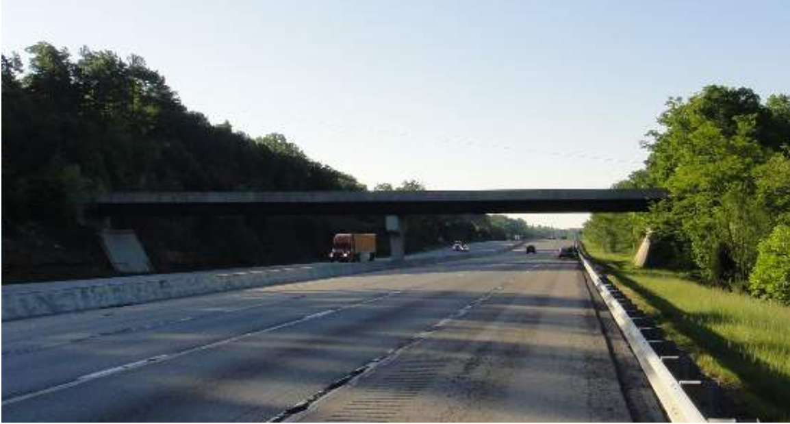
Figure 31. Vegetation Build-Up Around Abutments of I-75 Overpass Bridge
