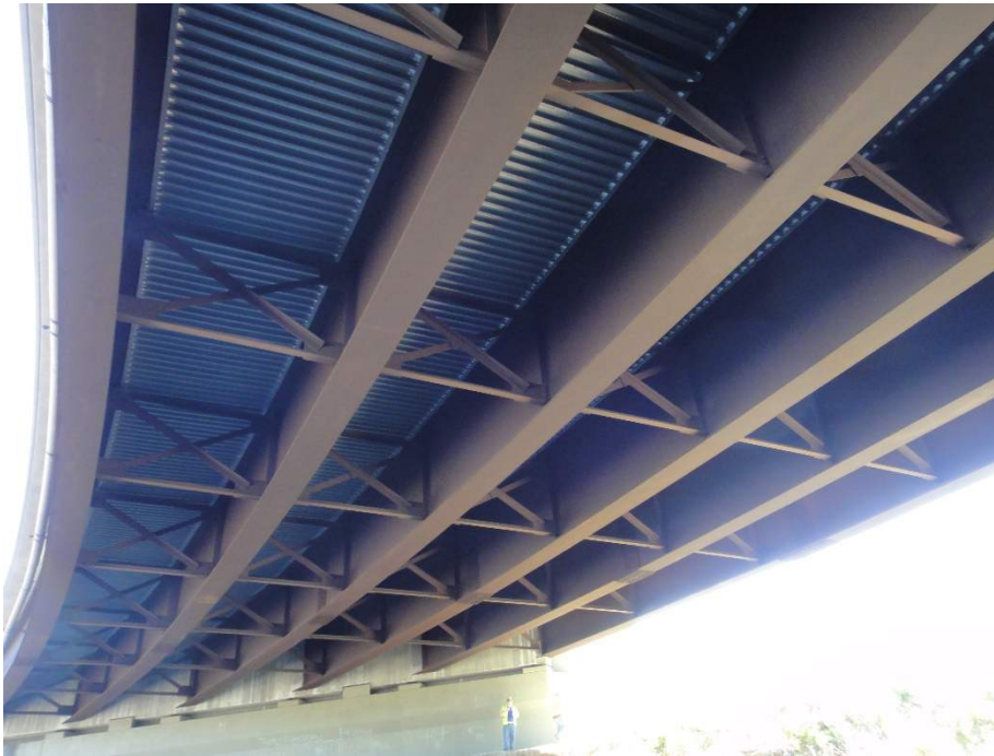
Figure 1. Deck Girder Bridge Showing Proper Appearance of UWS Patina
