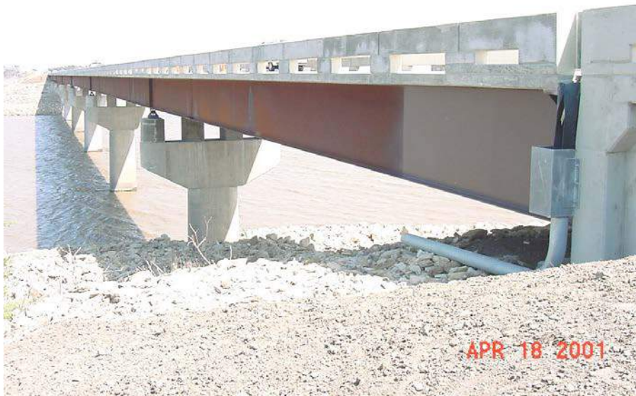
Figure 17. Kansas DOT UWS Girder Painted About 25 Feet from Beam End
