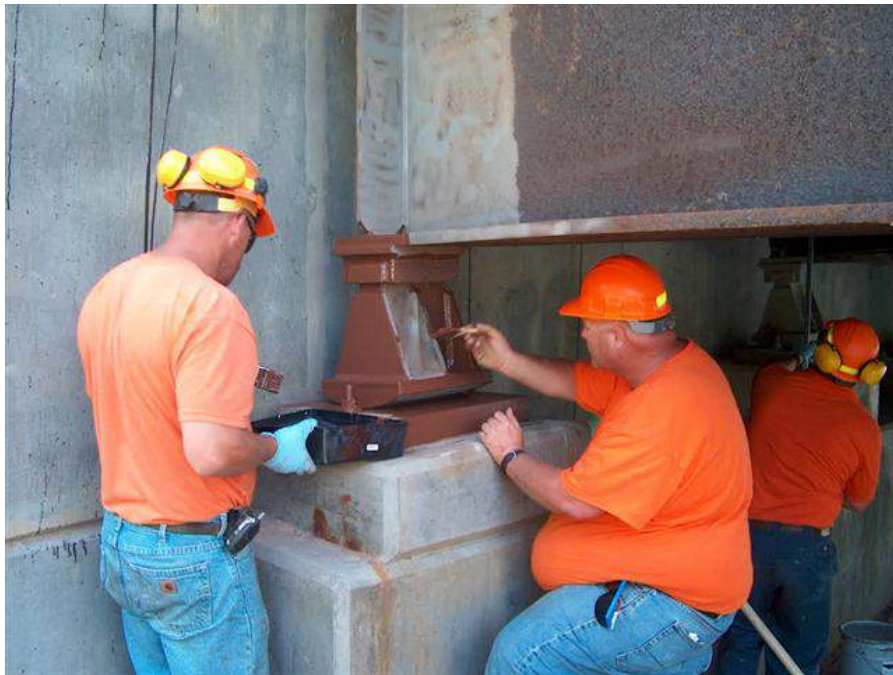
Figure 14. New York State DOT Maintenance Personnel Painting UWS under Deck Joint
