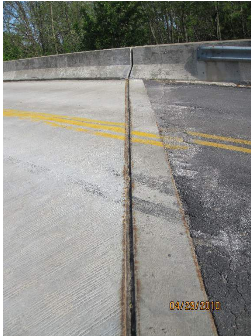
Figure 22. KY 1893 Bridge Deck with New Overlay and Deck Seals
