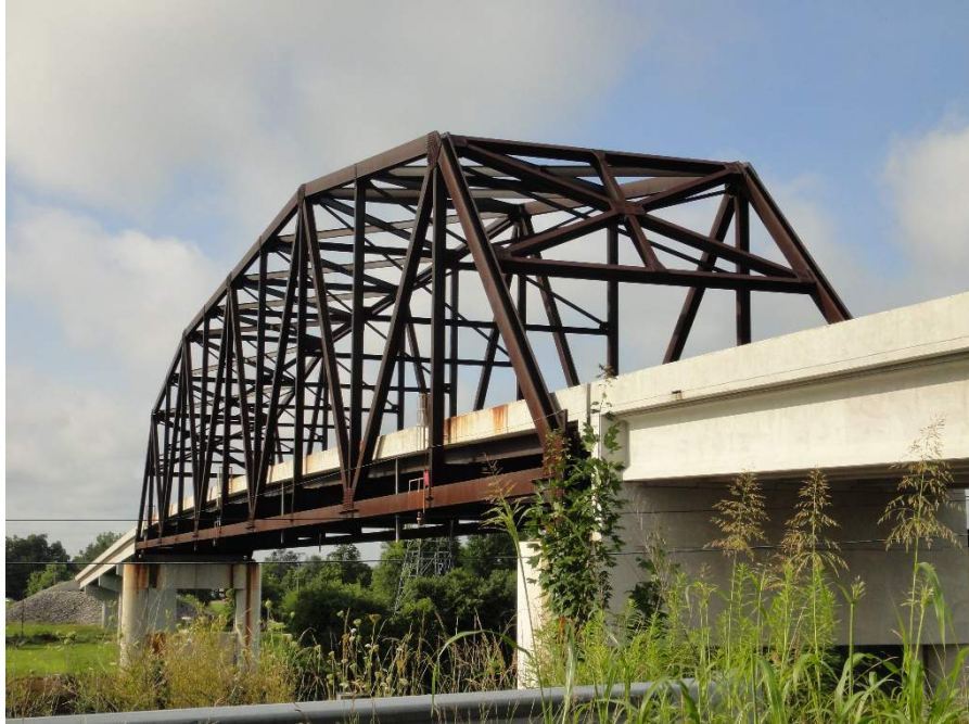
Figure 19. KY 81 UWS Truss over Green River at Calhoun, KY
