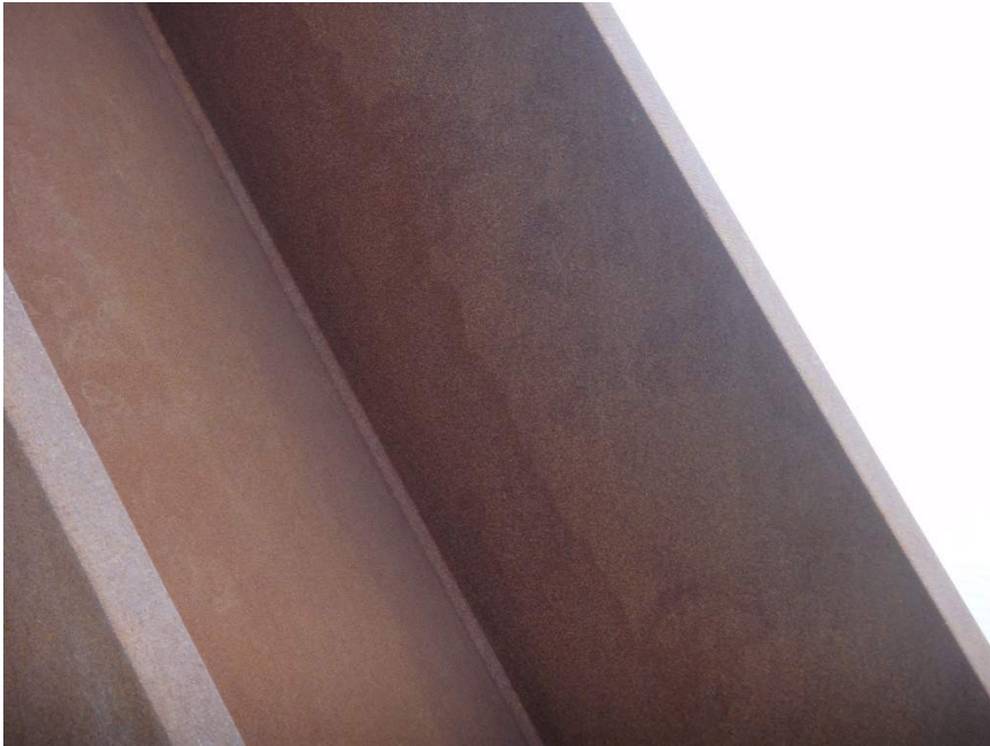
Figure 6. Topside of Same Diagonal Opposite Location Shown in Figure 5
