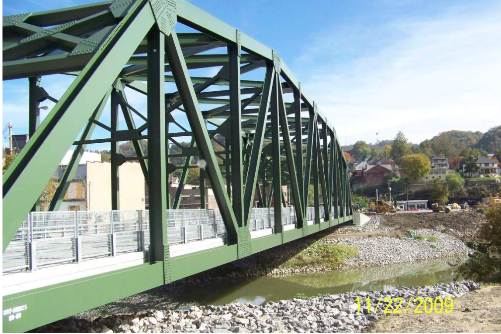
Figure 29. Painted Truss Employing Weathering Steel – KY 451 over North Fork of Kentucky River
