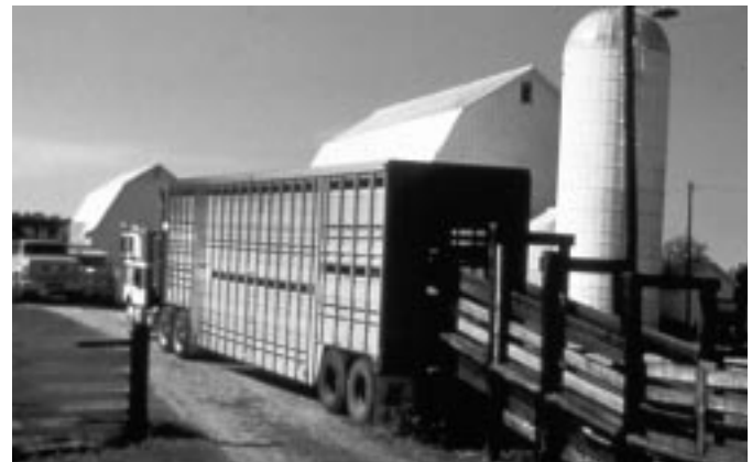
Figure 13. Sloped wooden loading chute without solid sides.
