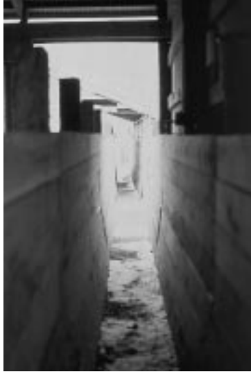
Figure 3. Undesirable working chute where cattle face bright sunlight.
