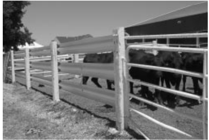
Figure 15. Holding pen with sidewall made from guardrail.
