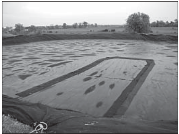
Figure 6. Opening for the access of agitation and pumping equipment in a geotextile-covered manure storage.
