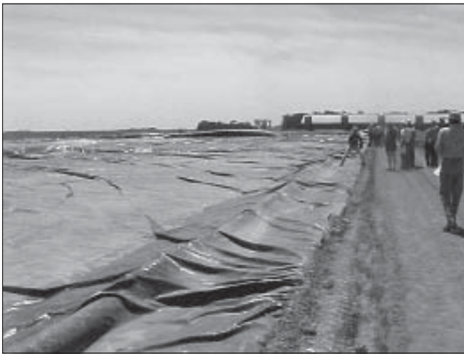
Figure 3. Anchor trench on impermeable plastic installation.
