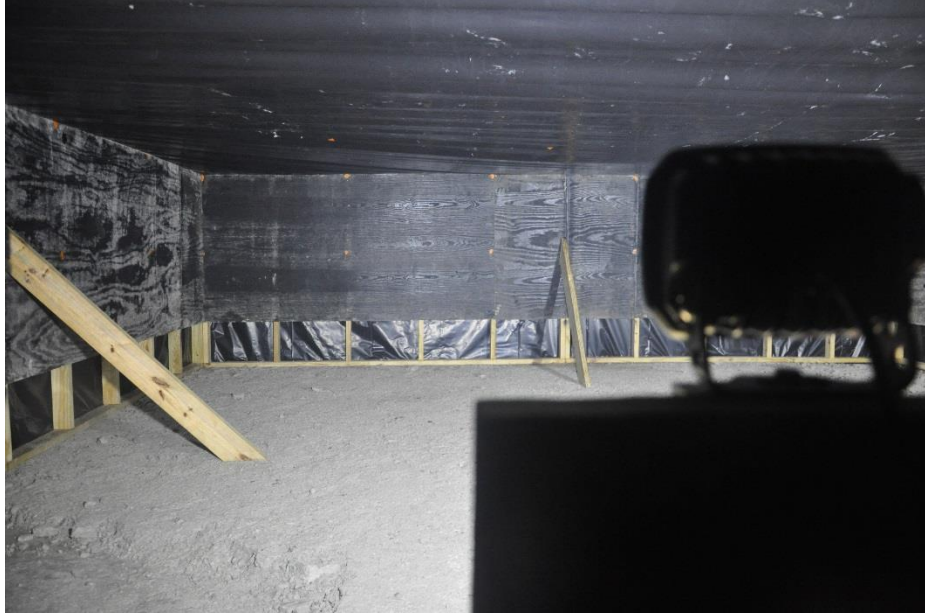
Figure 3.8: Example light setup (roof bolt machine operator perspective)
