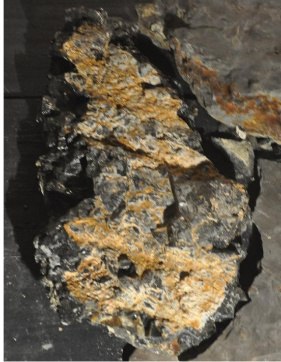
Figure 4.24: Coal Roof Using Halogen Euro Beam Pattern
