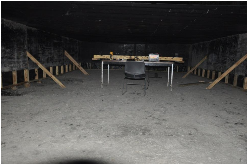
Figure 3.2: Recreated Entry (interior)
