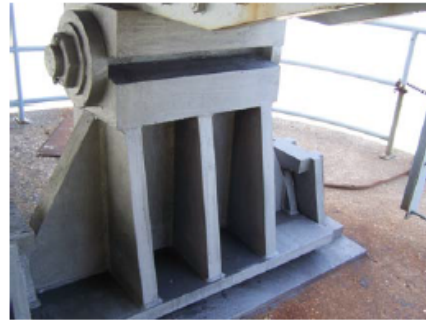
After Cleaning and Grease Application
