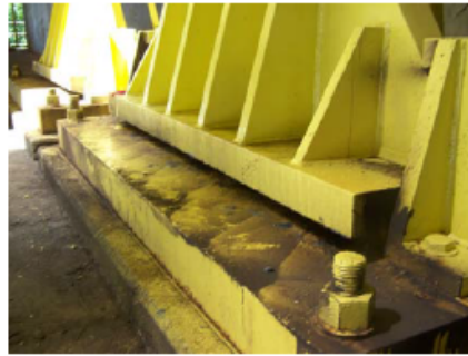
Before Cleaning and Grease Application
