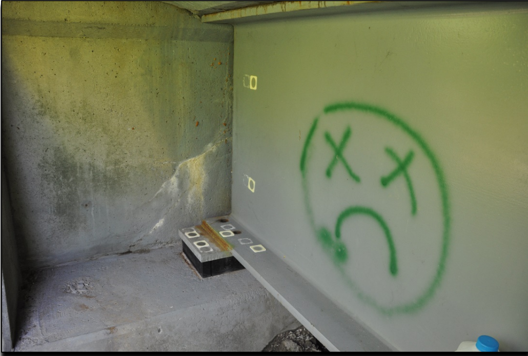
Figure 14. Conductivity tests location on a beam end after bridge pressure washing.
