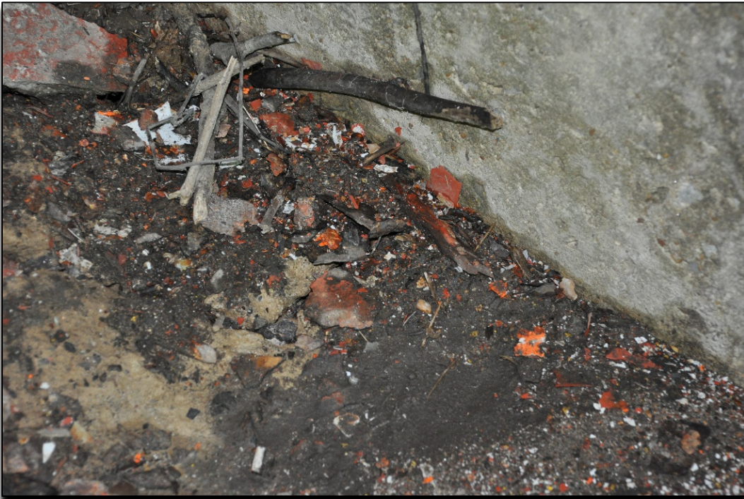
Figure 7. Paint Left on the Ground after a Bridge Washing Operation
