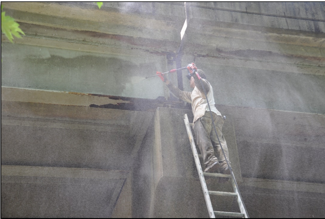
Figure 9. Worker on Ladder Washing Beam Ends
