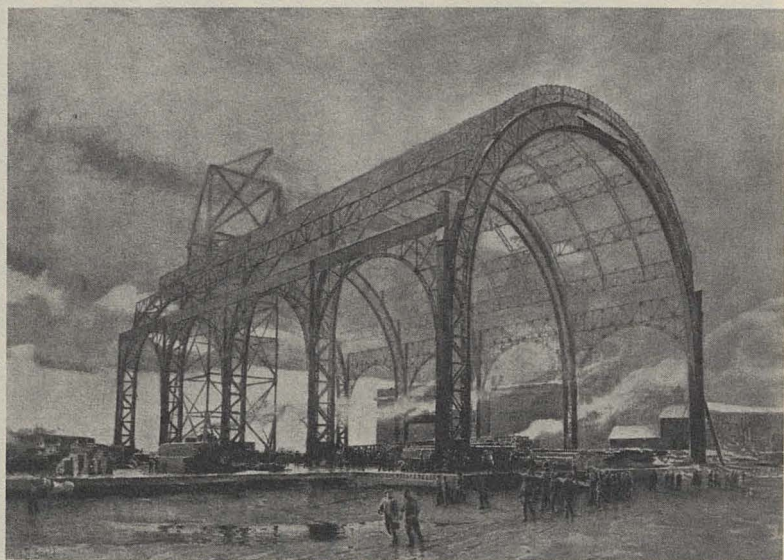
Fig. 11 The Trusses of the Machinery Building—World's Columbian Exposition of 1893
