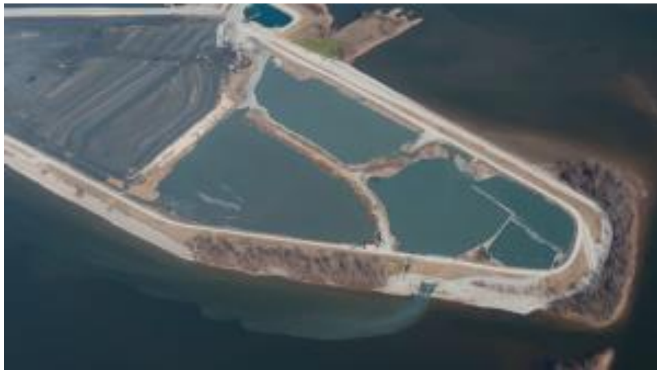
Figure 1.8: TVA's Johnsonville power plant impoundment (Southern Alliance for Clean Energy, 2013)
