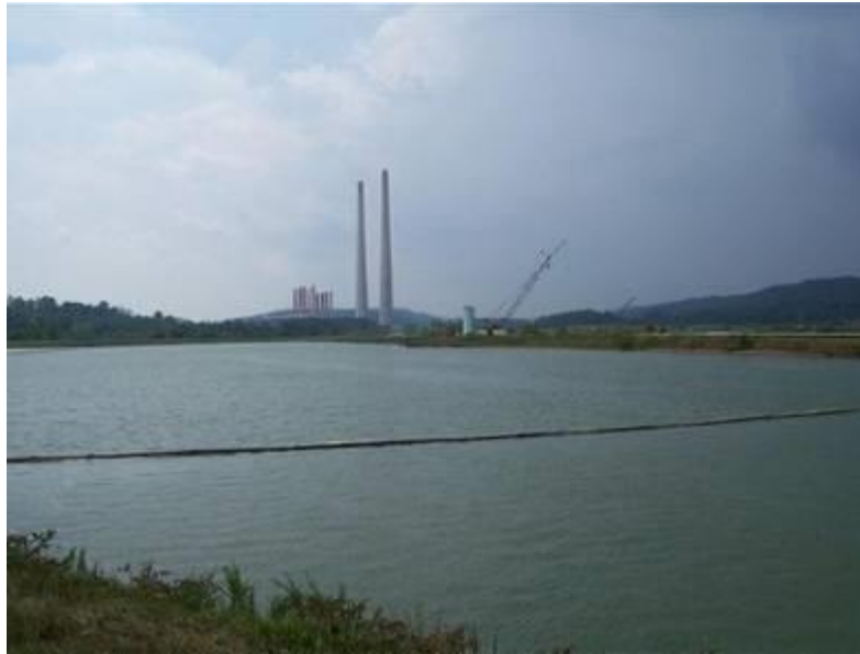
Figure 1.18: Kingston Plant coal ash retention pond two years before the December 2008 failure (EPA, 2009)
